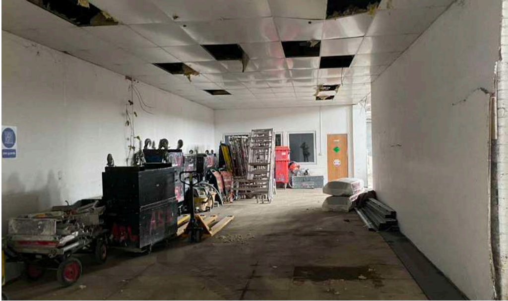
View 9- Inside of the existing building
