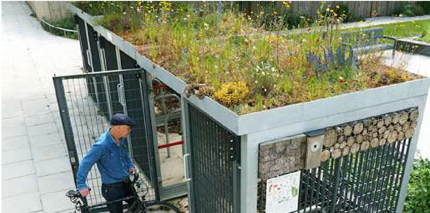
Bike store with integrated green roof and bug hotels
