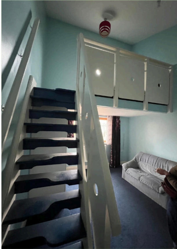
View 10 - View of alternator stair access to bed deck
