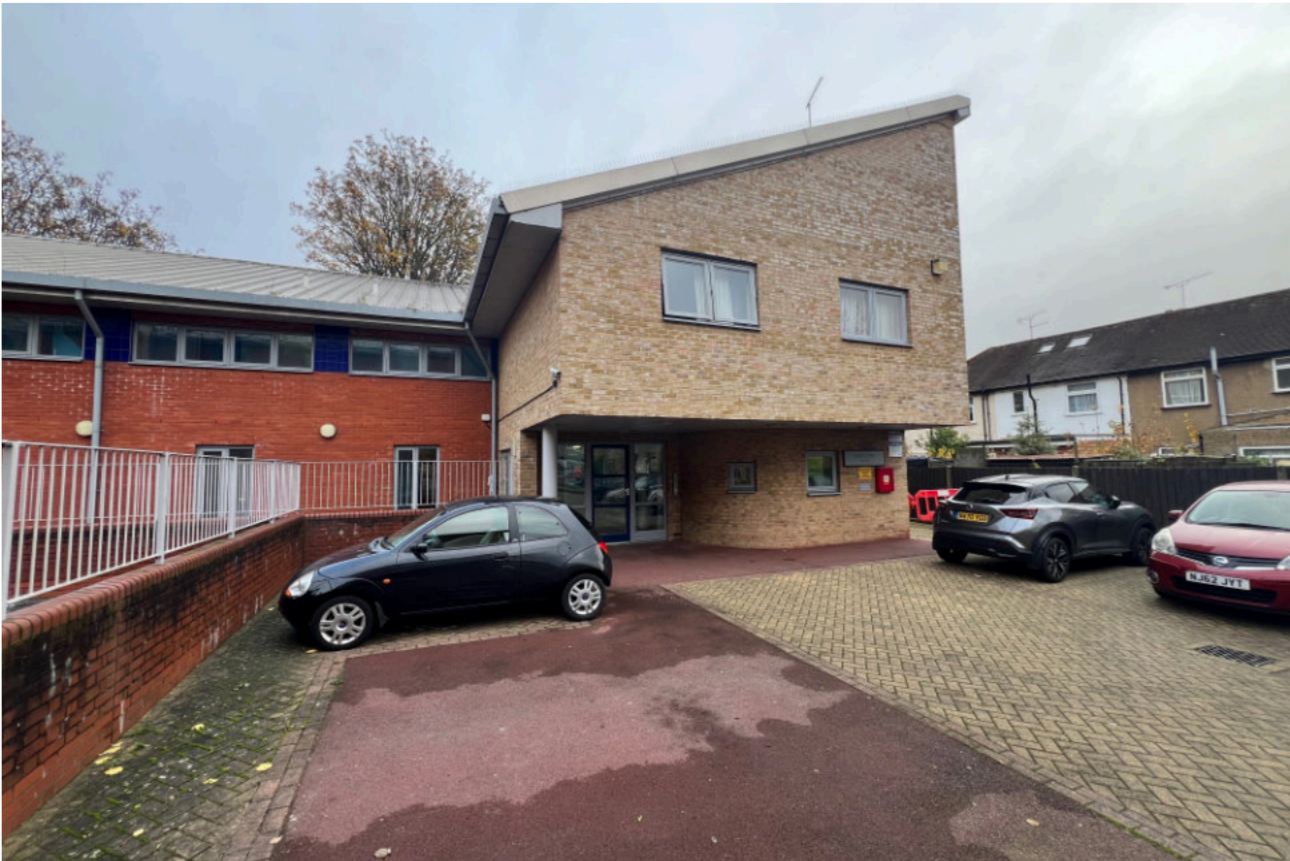
View 04 - View looking towards the communal entrance
