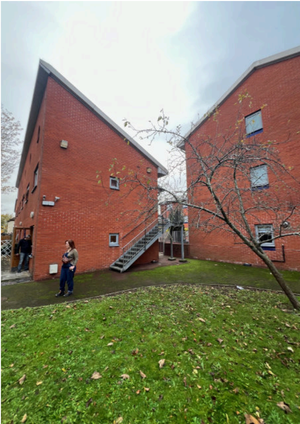
View 06 - View looking at west corner assisted living block
