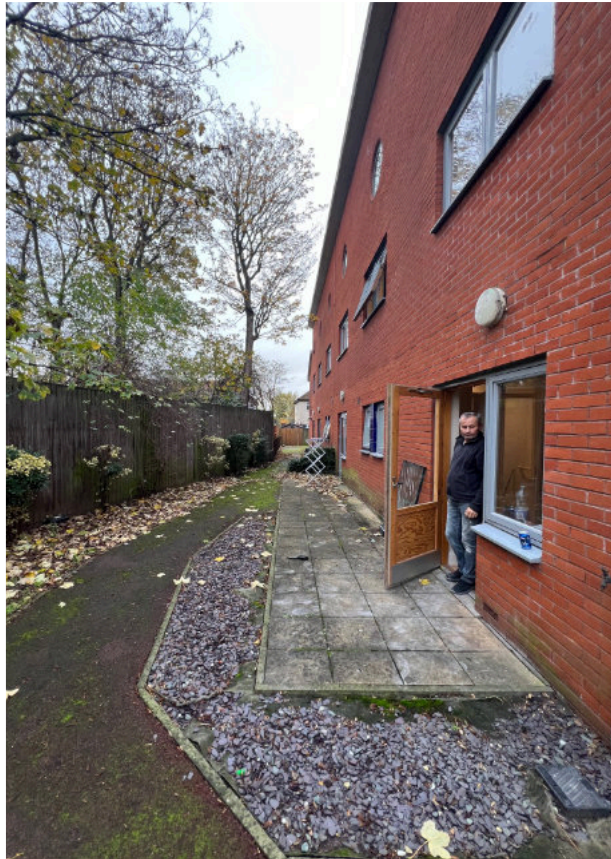
View 08 - View looking east along rear of assisted living block
