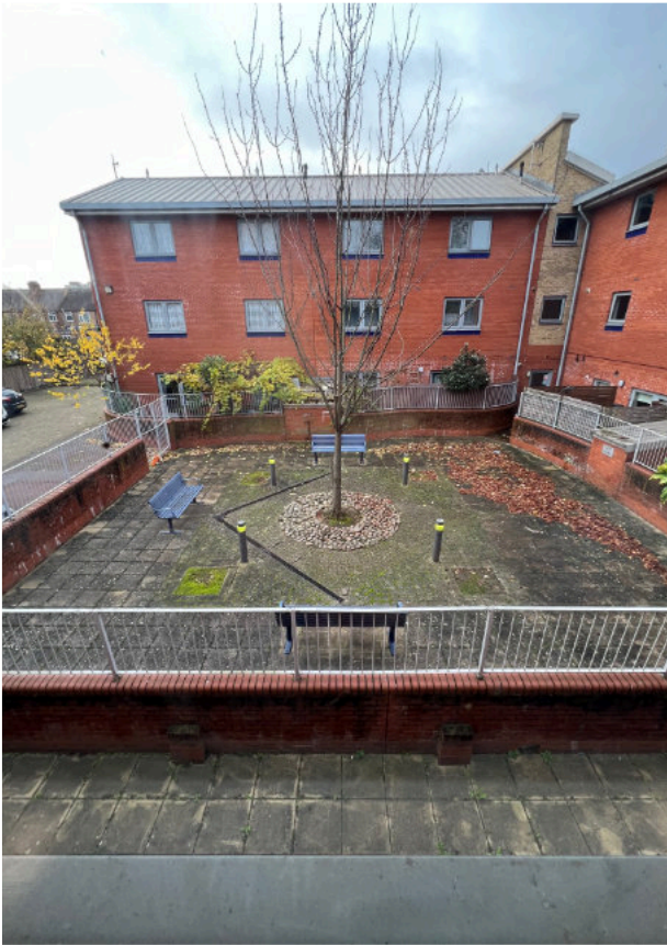
View 05 - View looking at courtyard from first floor
