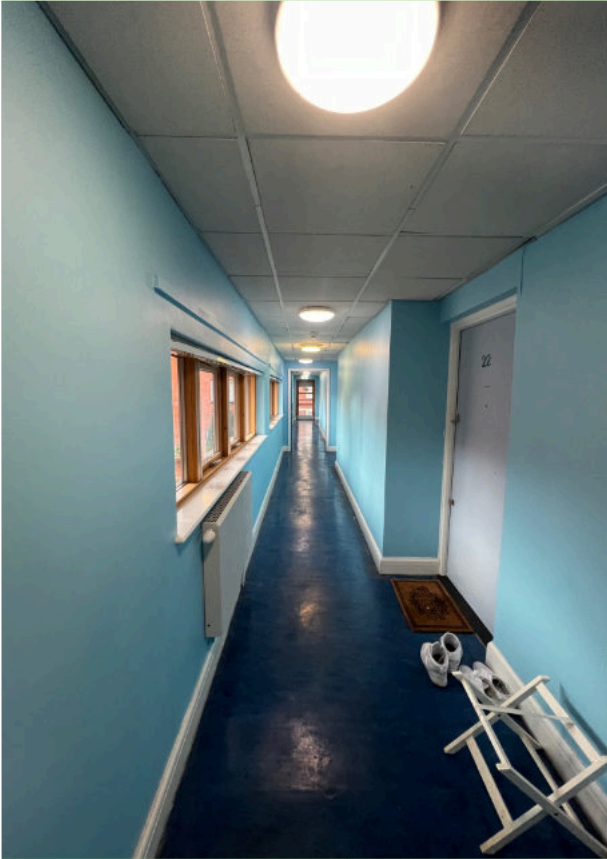
View 10 - View of bed sit access corridor
