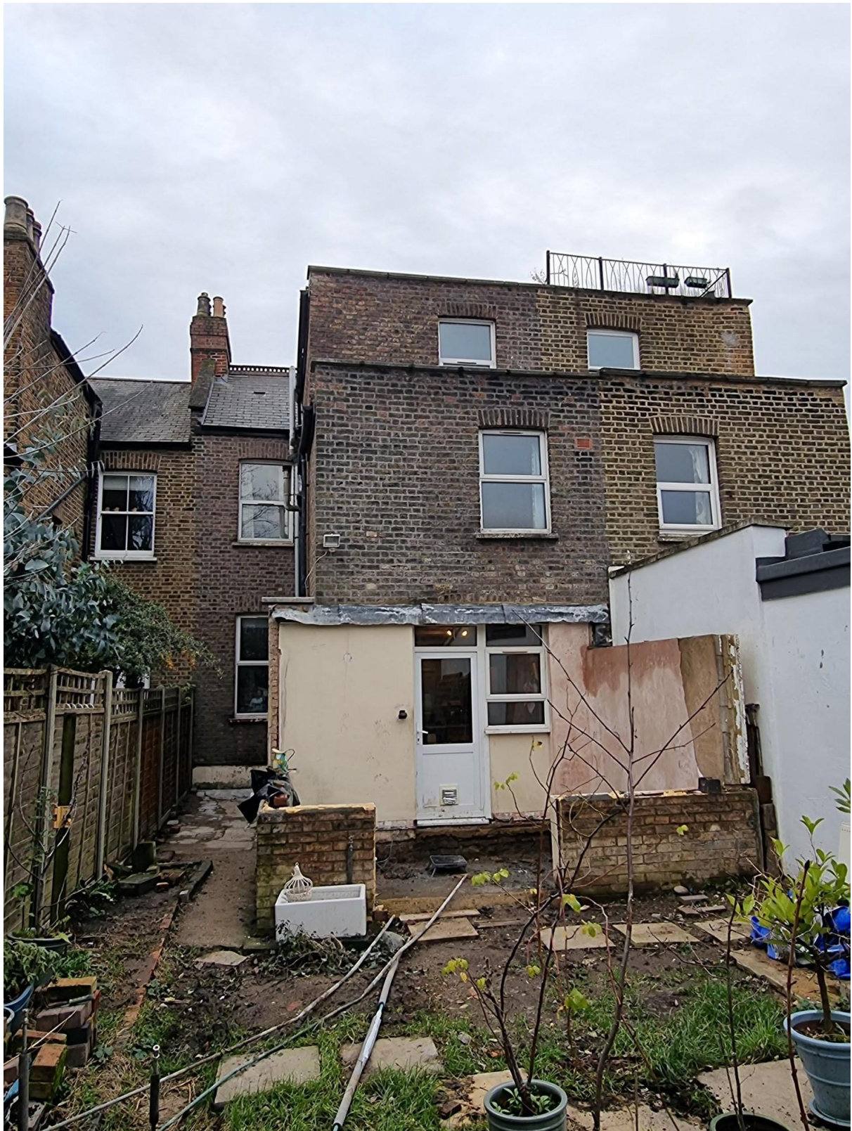
Rear of application site
