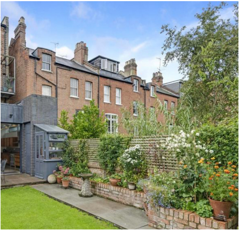
64 and 68 Langdon Park Road
