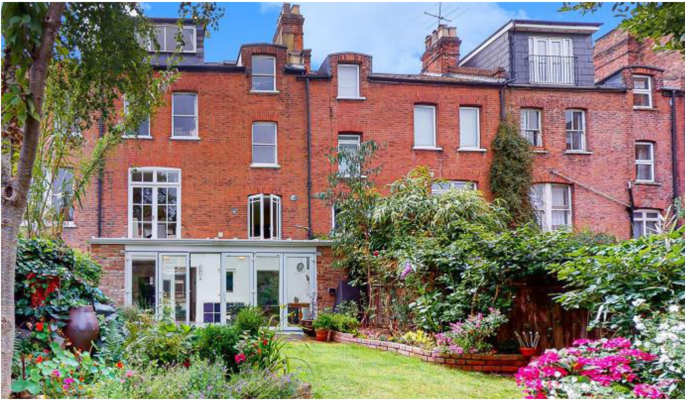
64 and 68 Langdon Park Road
