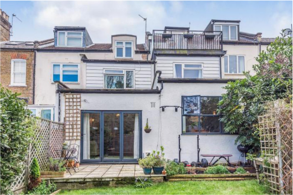
7 and 9 Langdon Park Road
