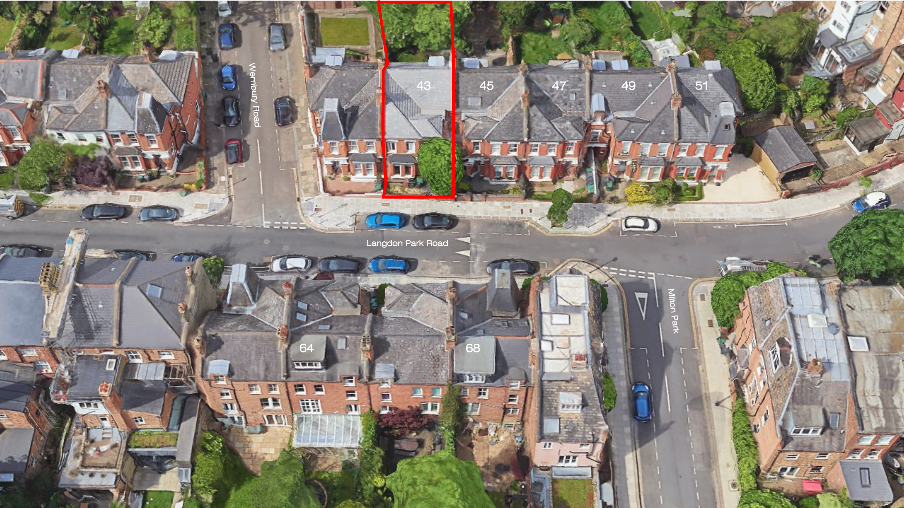
View of dormer windows at 64 and 68 Langdon Park Road, and of rooflights at 64, 68, and 45 to 51.
