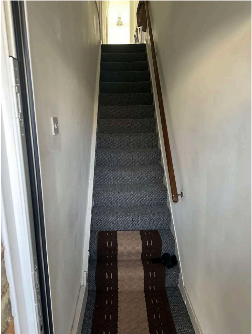
Image of the internal staircase to be removed
