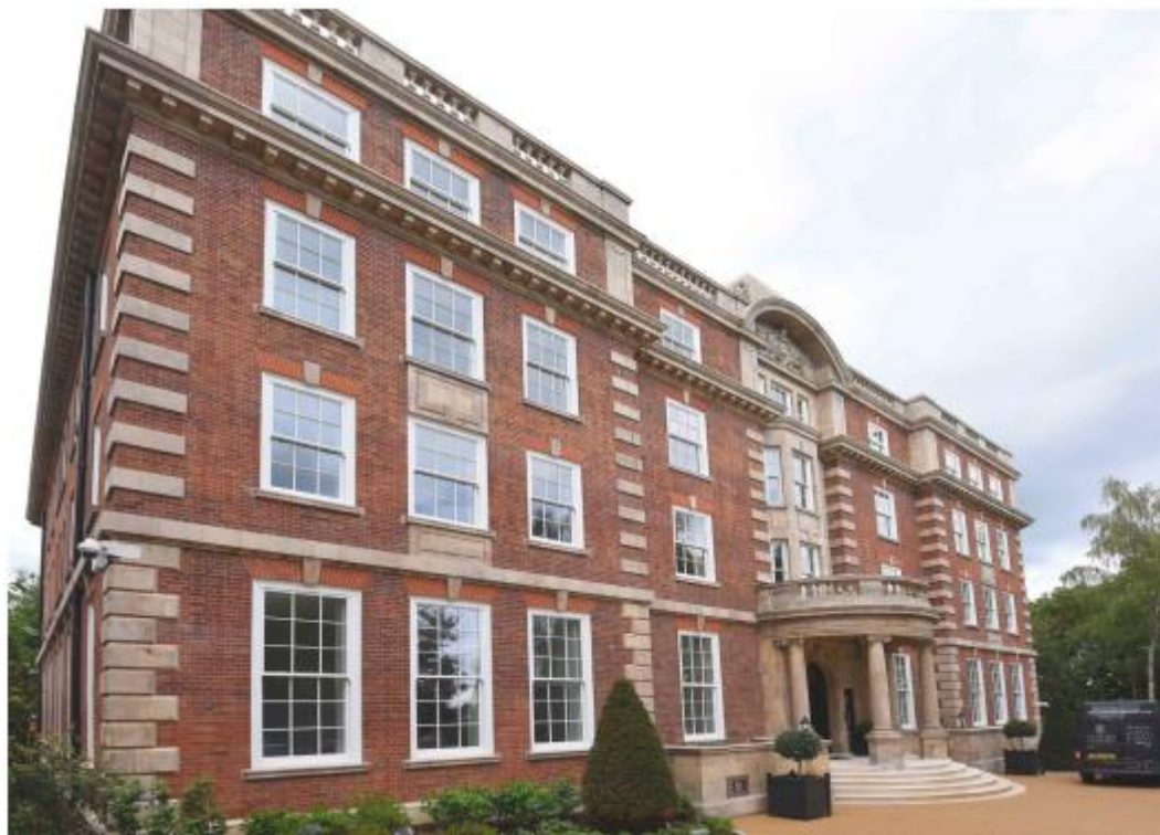
Figure 4.1 Furnival House, the principal frontage
