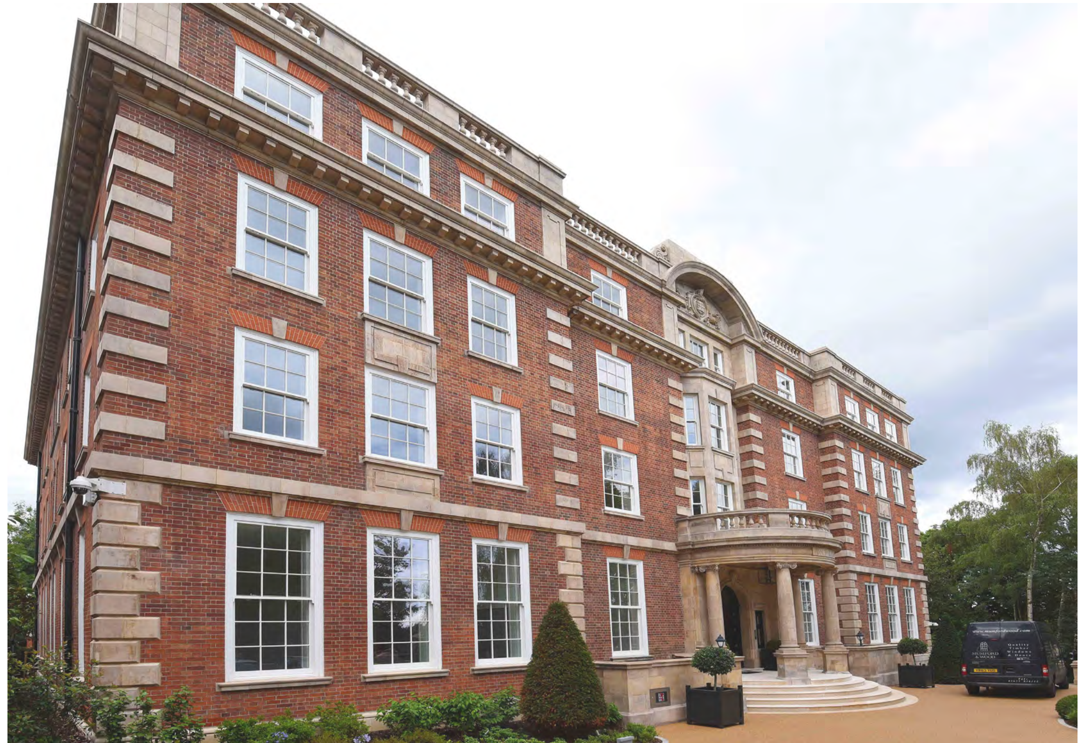
Photo of the front elevation of Furnival House
