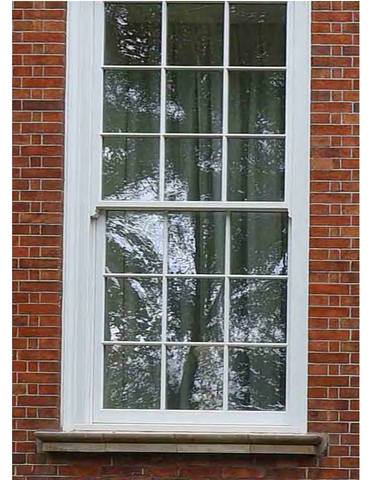
Photo of an existing window on Furnival House
