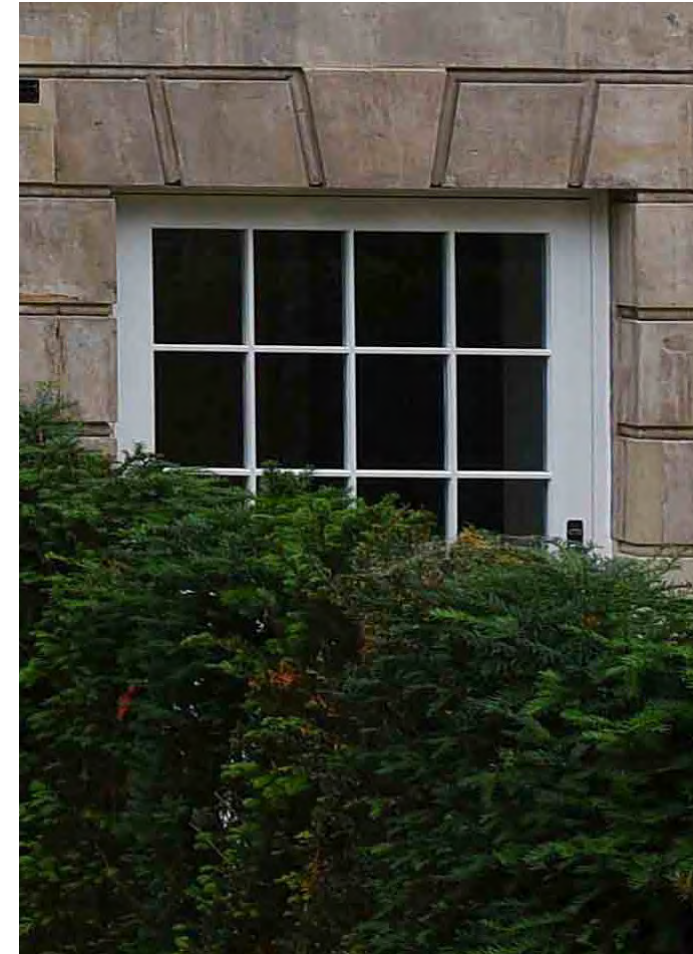
Photo of an existing door on Furnival House
