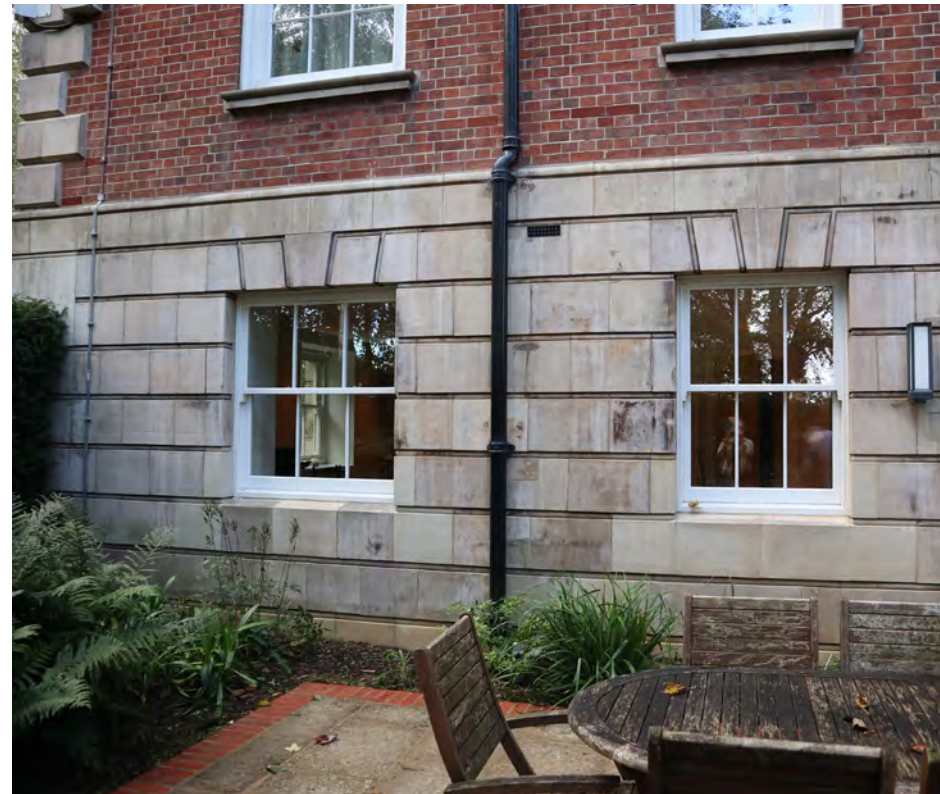
Photo of the existing windows.
