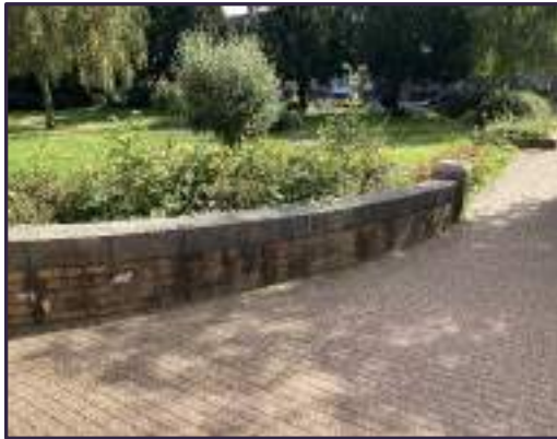
Figure 29 – External lighting located with blockwork wall
