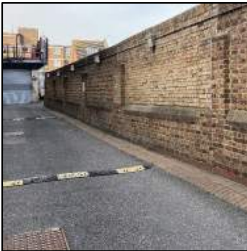
Figure 20 – Speed bumps and manhole covers
