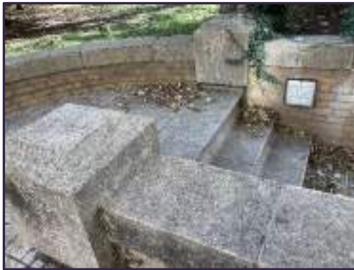
Figure 27 – External lighting located with blockwork wall
