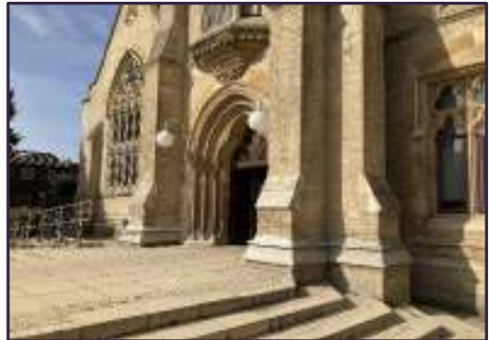
Figure 28 – External lighting located at front entrance of court
