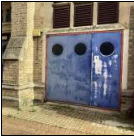
Figure 14 – Access to plantroom via external blue doors of courts
