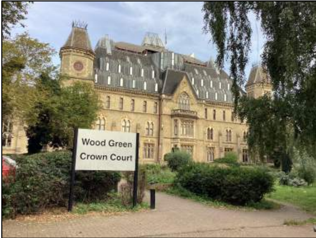
Figure 1 – External view of court building
