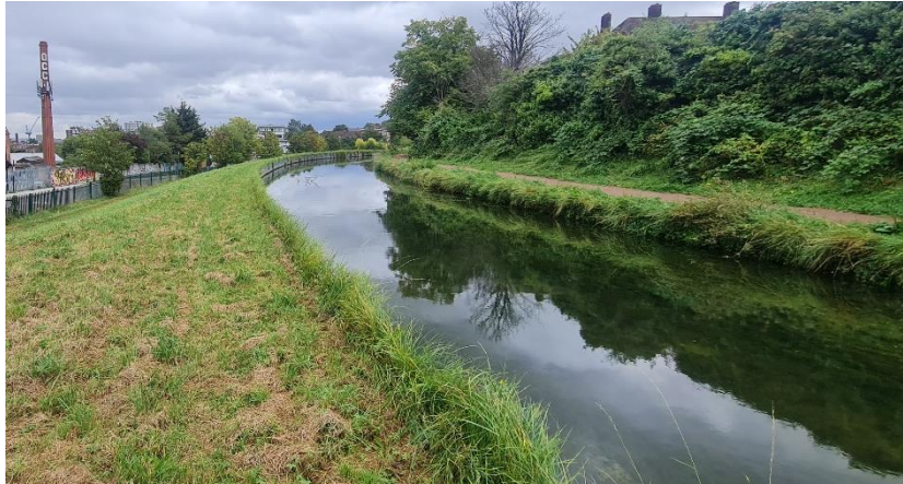
Plate 1: Canal piling along river banks
