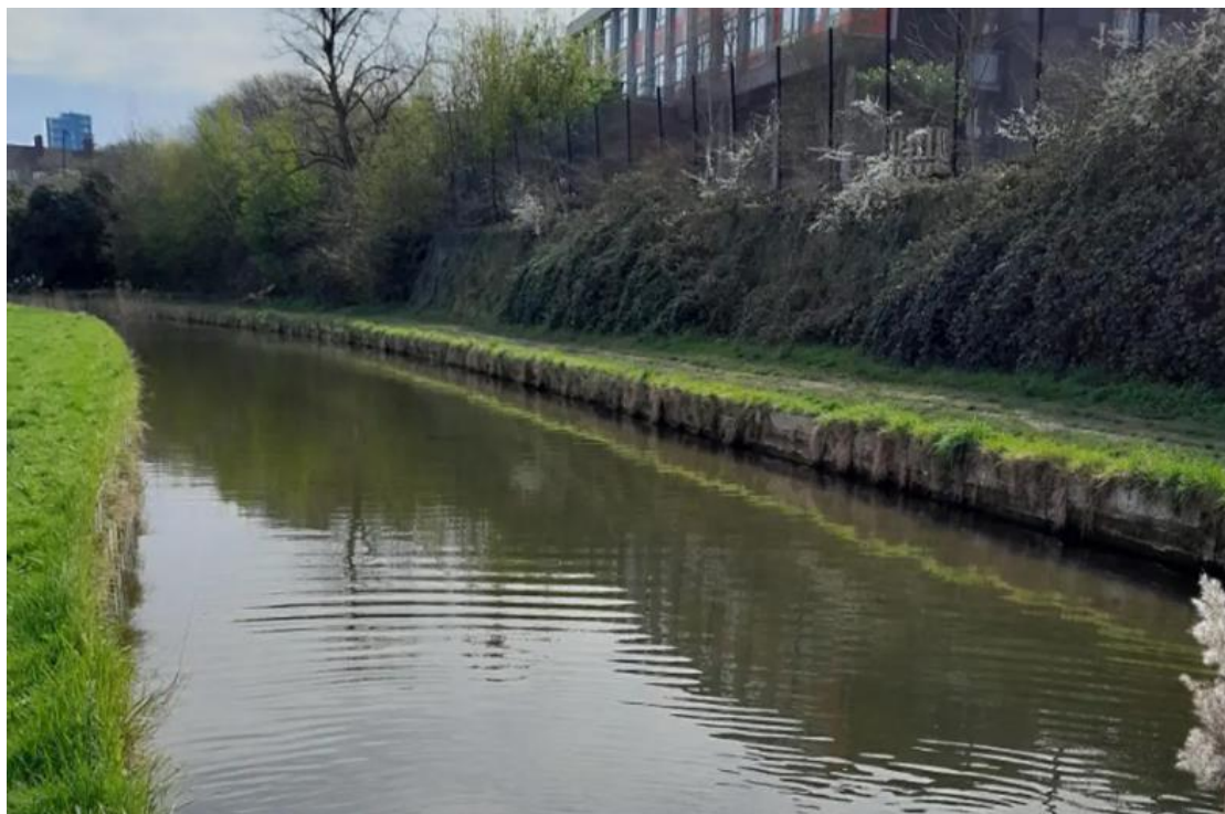
Figure 5: New River south of Eade Road (existing timber wharfing supported on 'H' piles on south bank).
