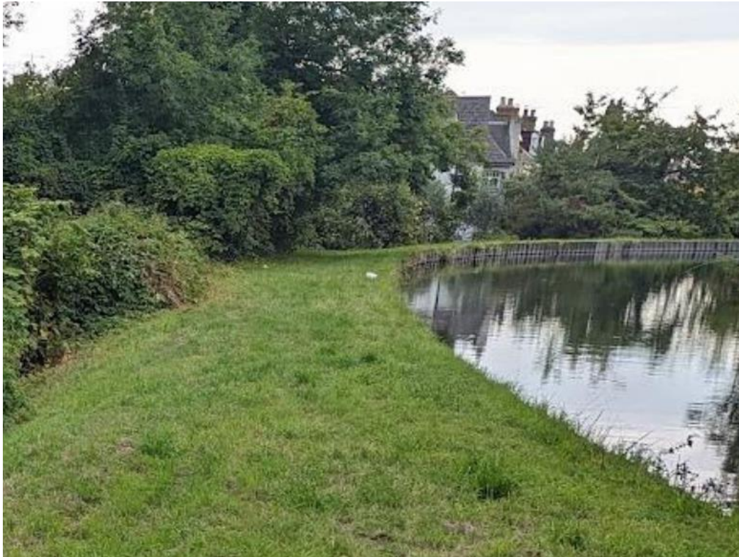
Figure 6: New River south of Eade Road (existing sheet piling on north bank)
