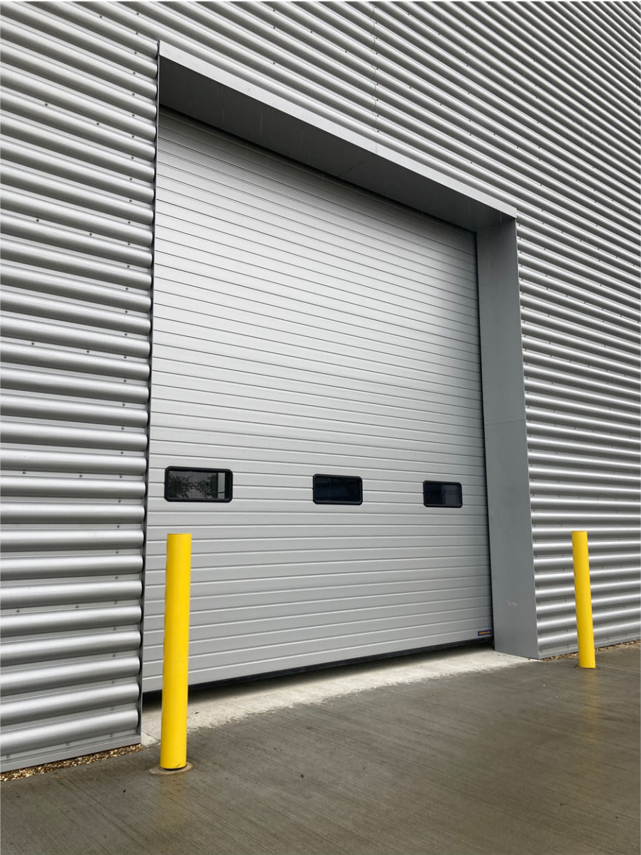
TYPICAL LOADING DOOR
