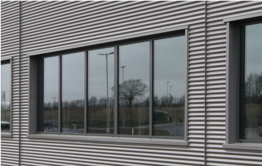
TYPICAL OFFICE WINDOWS
