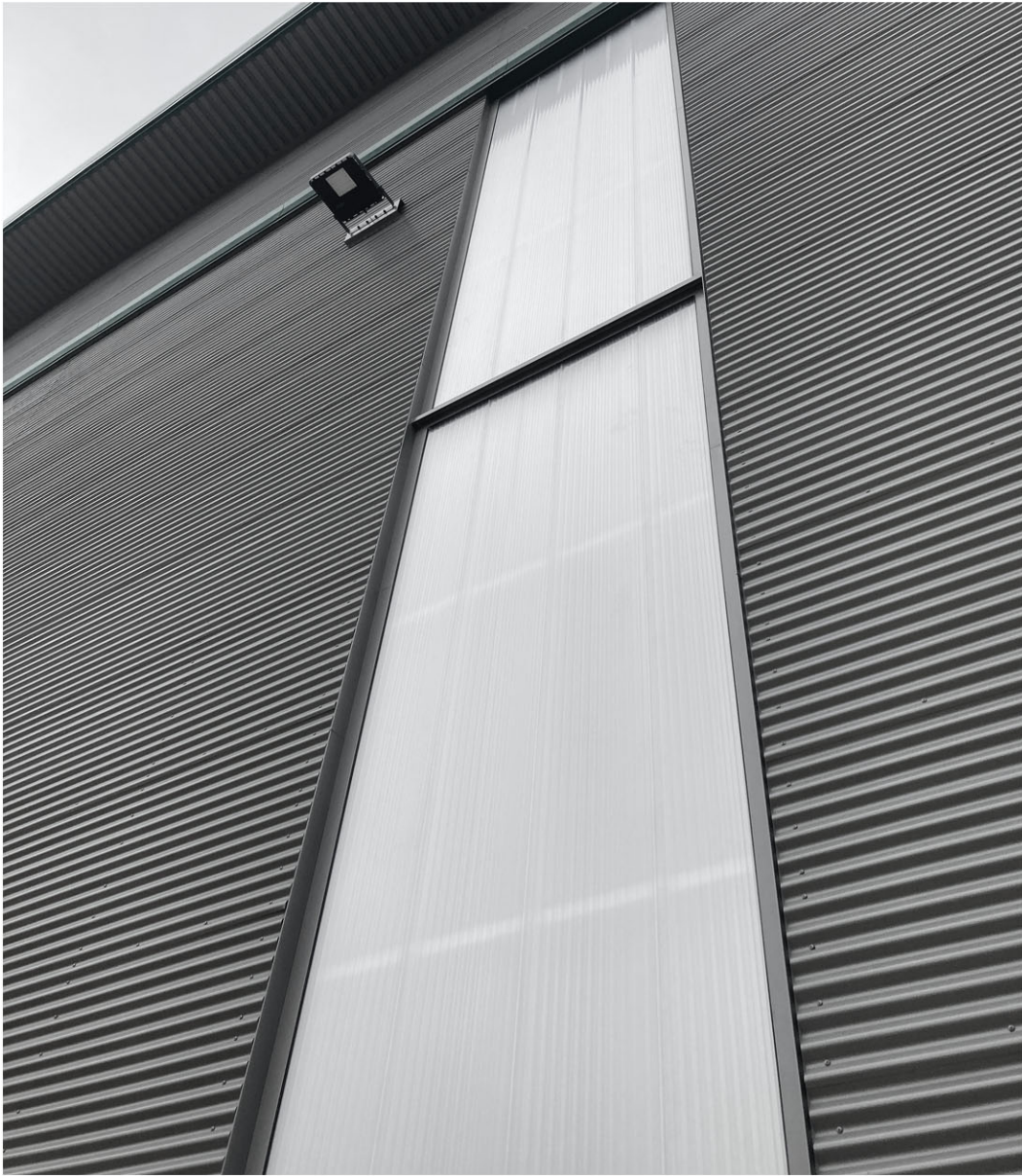
TYPICAL TRANSLUCENT GLAZING SYSTEM
