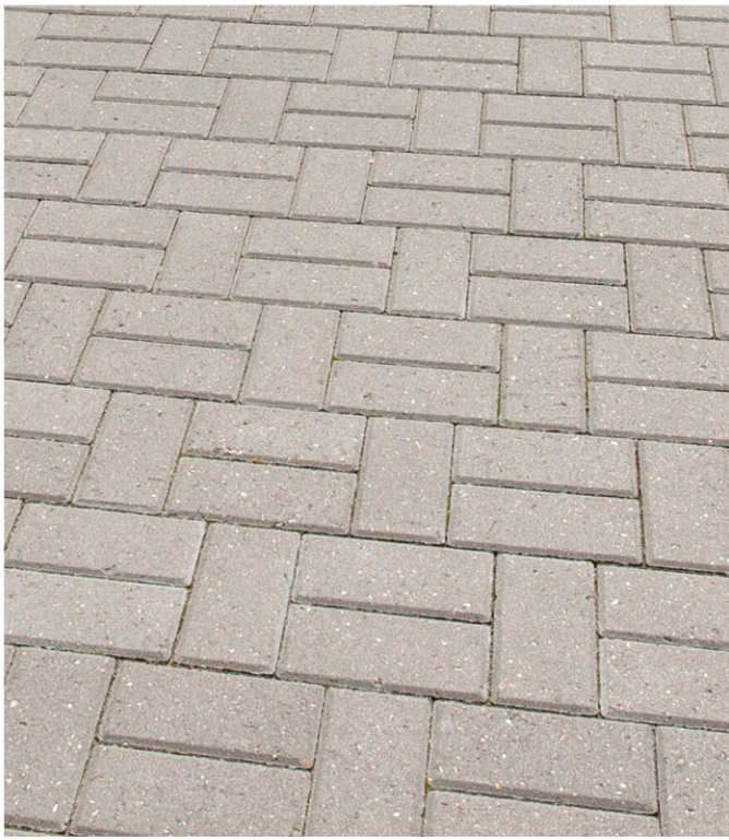
CONCRETE BLOCK PAVING TO FOOTPATHS
