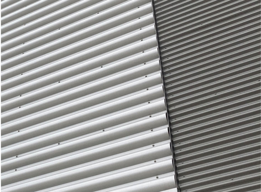
TYPICAL CLADDING JOINT
