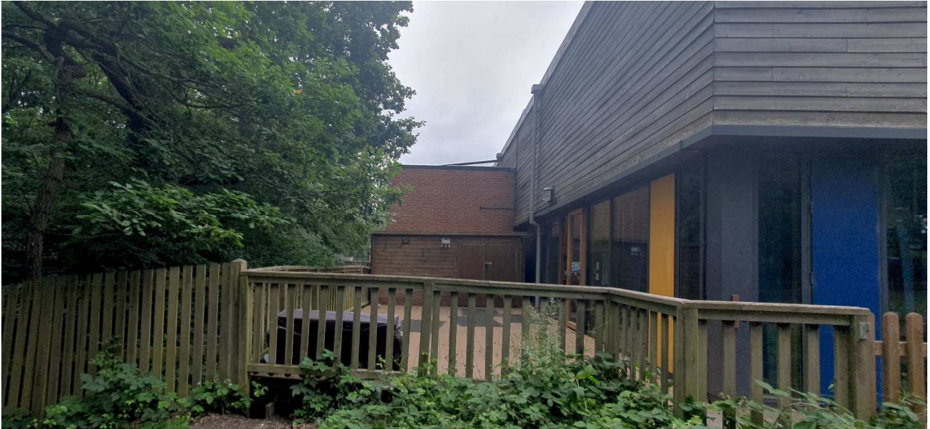
1 Terrace and Storage Shed - view looking North-West
