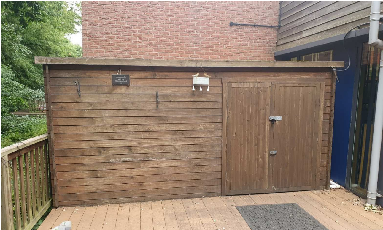
4 Storage Shed close-up
