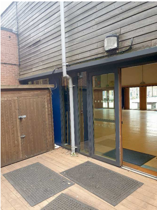
2 Main Hall and timber shed Storage - view from the Terrace
