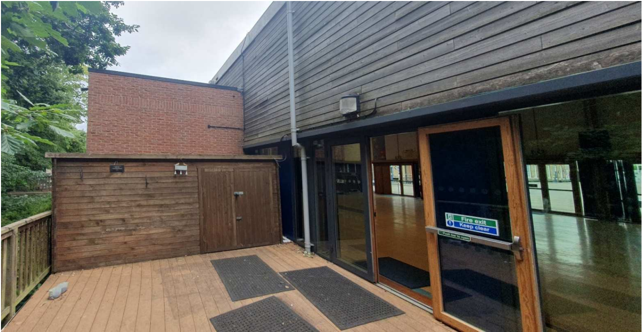
3 Storage Shed - view looking North
