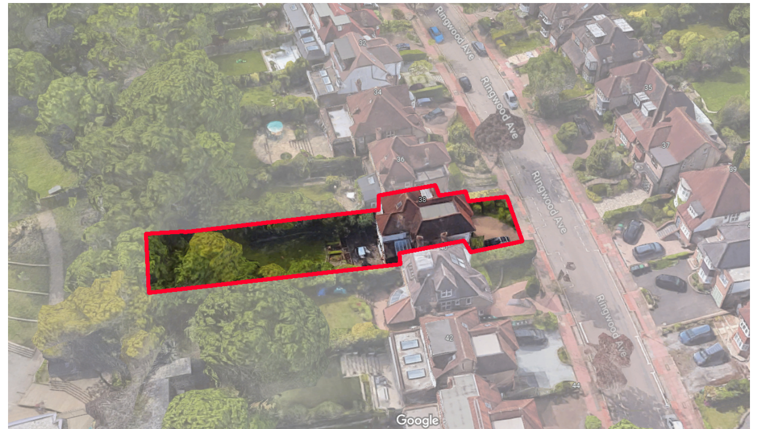
2. Birds eye view to rear of No.38 Birchwood (looking South).
