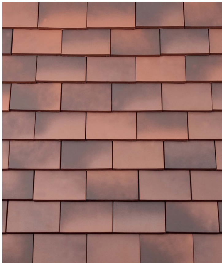
1. Rosemary red clay plain tiles to main roof and dormer
