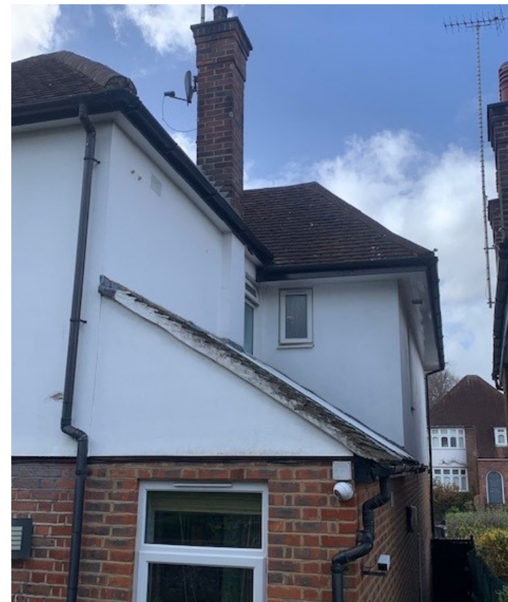
4. View from rear to side alley of No.38
