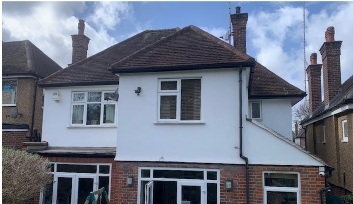
3. View of existing rear elevation from rear garden
