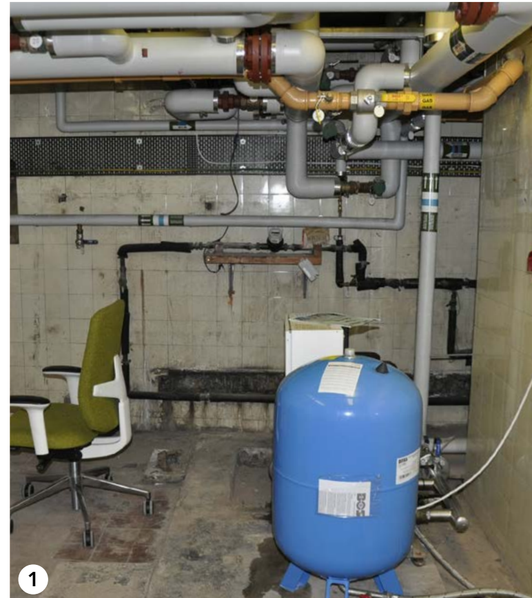
1 tiled floors and walls
