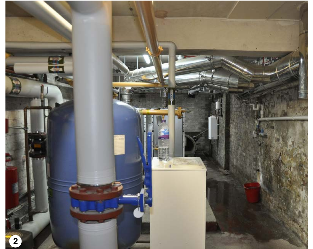
2 concrete floors, brick walls
