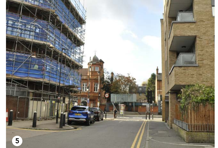
View of the 639 Enterprise Centre looking north from Hampden Lane highlighting the 2012 Gort Scott timber street facing addition
