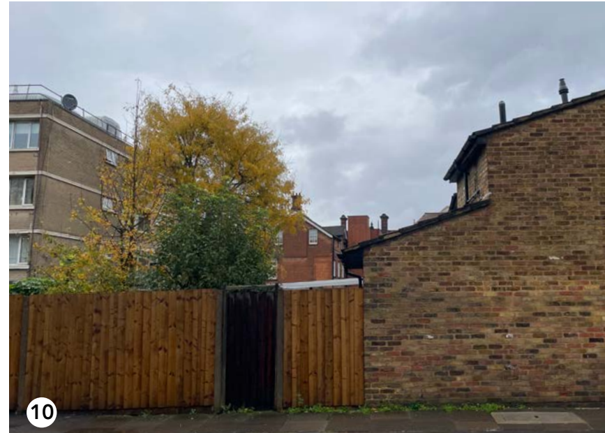
View of the 639 Enterprise Centre looking east from Pembury Road. End gable and lift tower are visible over garden fences
