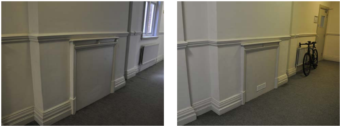
Historic fireplaces within south wing corridors at first floor with simpler surrounds
