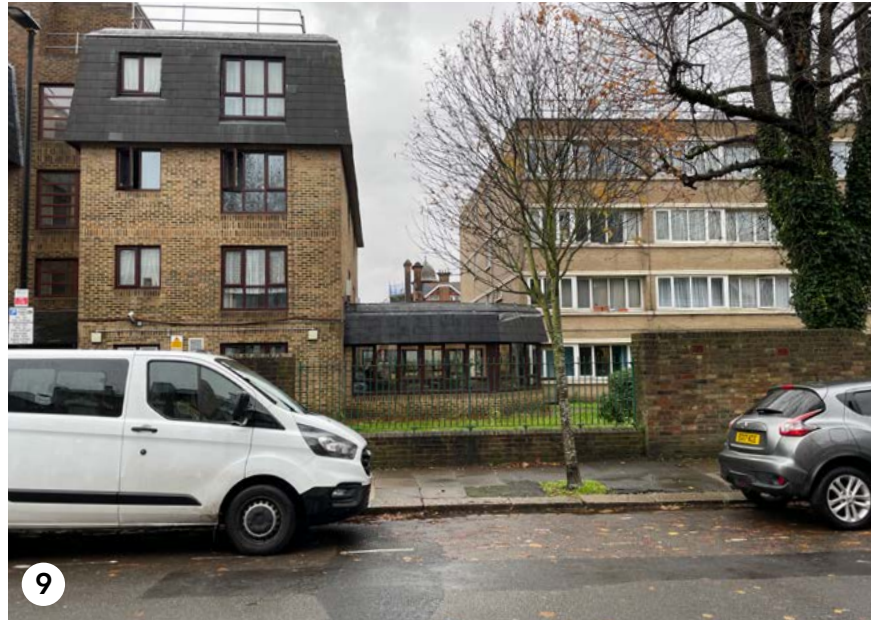
View of the 639 Enterprise Centre looking east from Pembury Road. The rear of chimney stacks and lantern are framed in the distance between modern housing blocks
