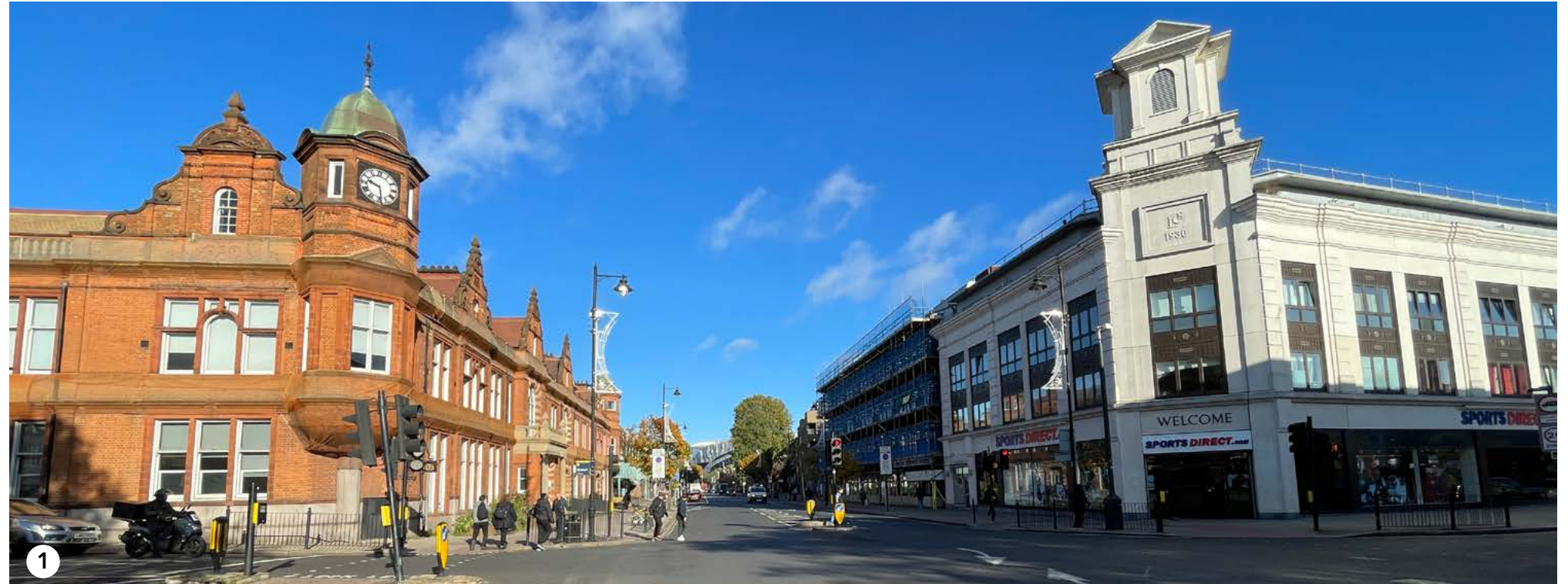
View along Tottenham High Road approaching 639 building, demonstrating its part of a pair of buildings forming an important gateway to the north of the High Road
