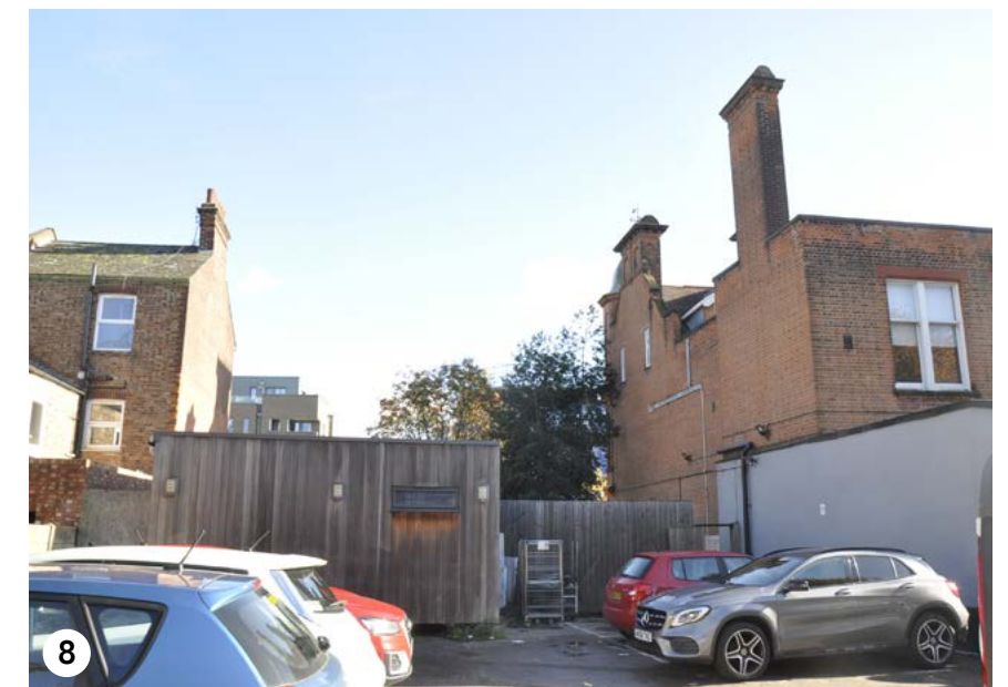
View of the 639 Enterprise Centre from the car park looking east. The north elevation sits opposite a line of terraced houses
