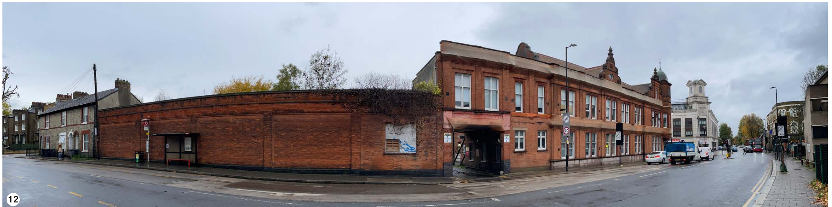
View of the 639 Enterprise centre looking north. The south elevation adjoins a monolithic red brick wall which is not part of the site ownership
