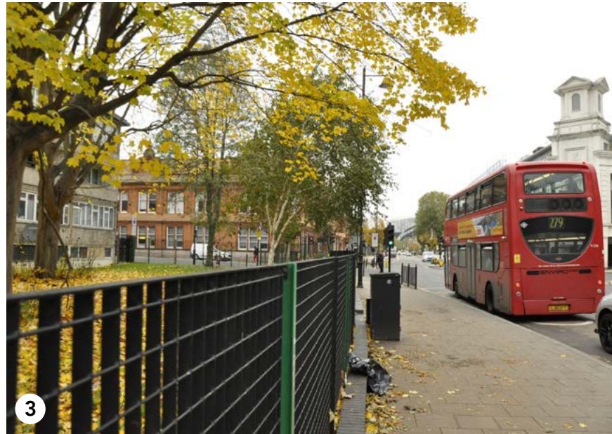
View of the 639 Enterprise Centre approaching from the south, the building is partially obscured by trees and the adjacent mid-late 20th century housing block, Millecent Fawcett Court
