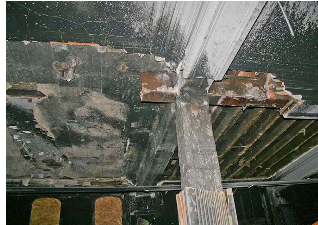
2012 - courtesy of Sergison Bates Architects
