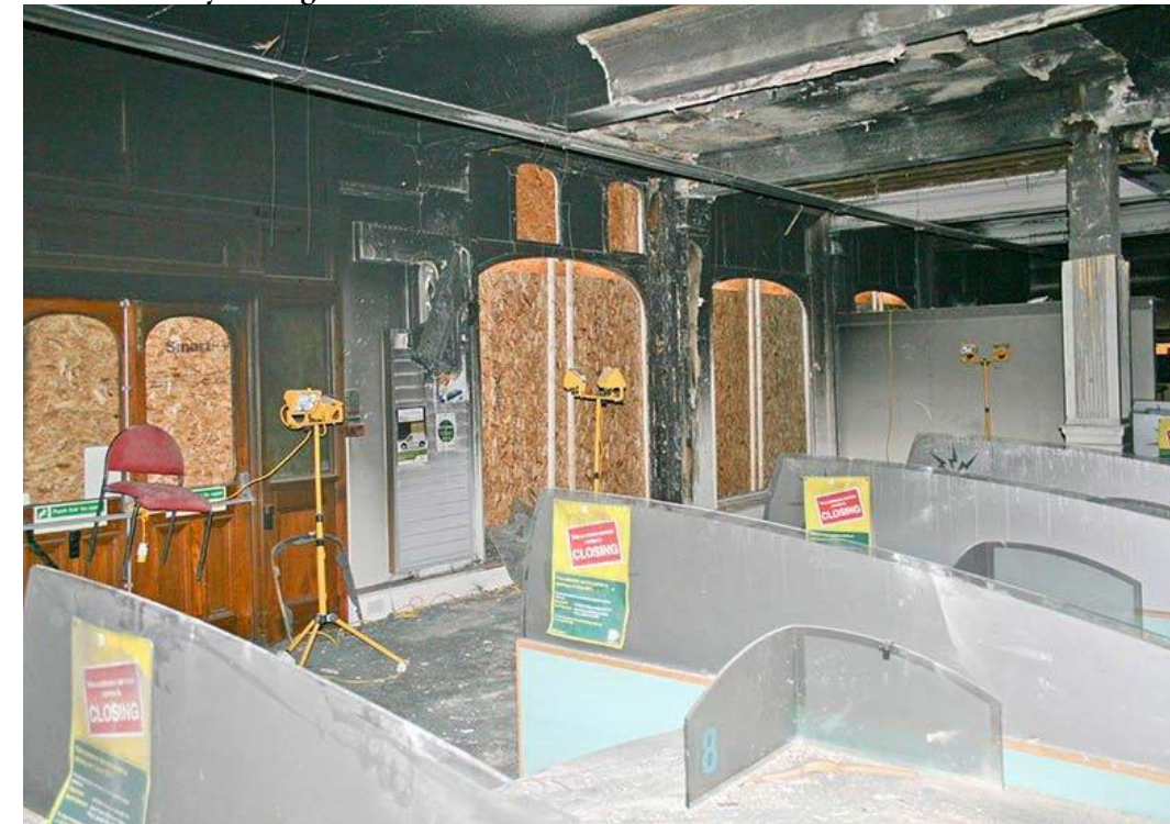
2012 - courtesy of Sergison Bates Architects
