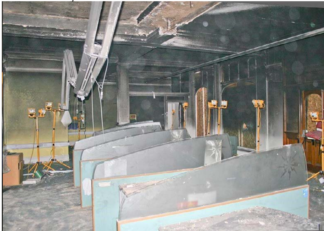
2012 - courtesy of Sergison Bates Architects
