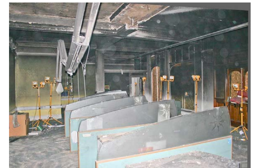
Charring to the building fabric after the 2011 riots image courtesy of the Trampery
