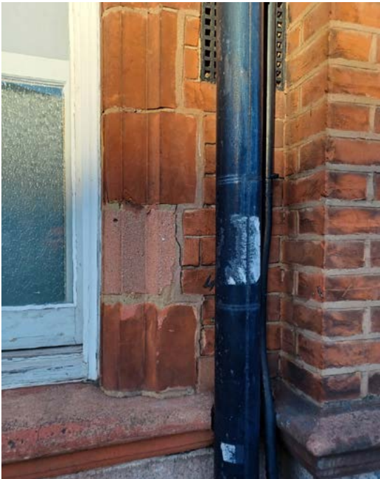
Inappropriate repairs
