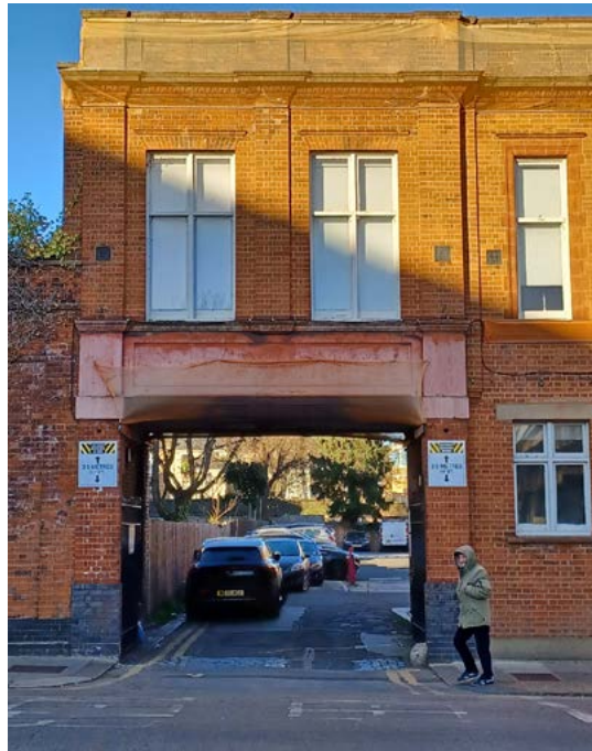
South elevation entrance to rear of building
