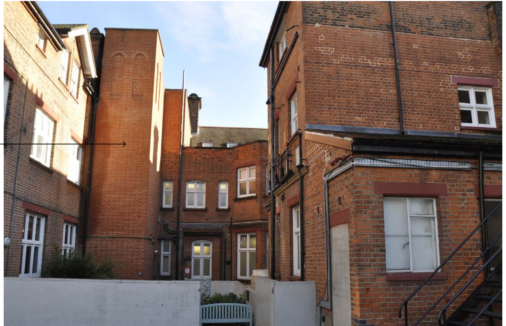
West elevation - modern brick lift tower as existing
