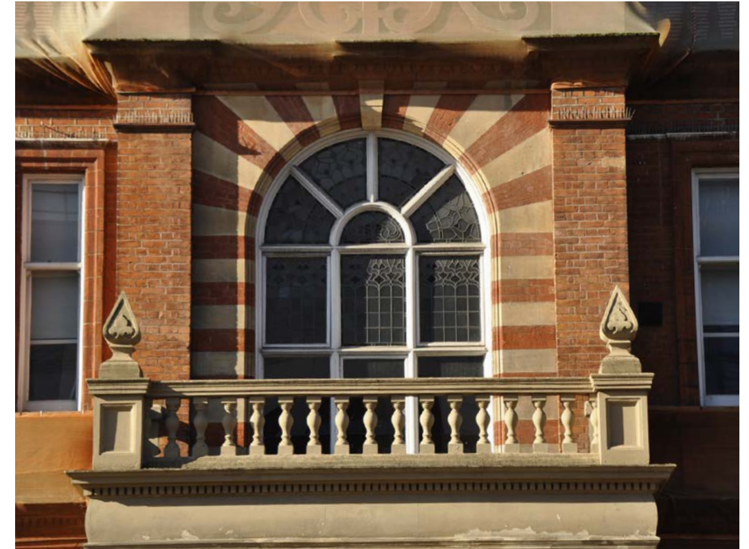
stained glass window to east facade
