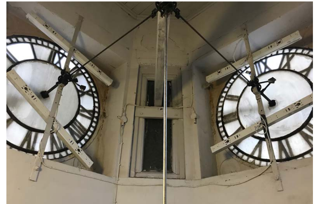
inside the clock tower
