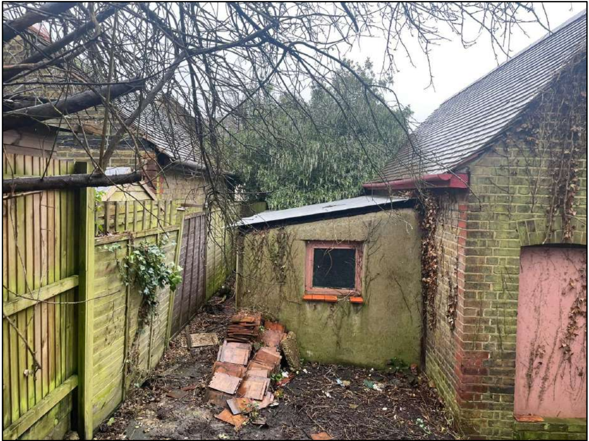
Photograph 5 – Photograph taken of the rear of the structure on site.
