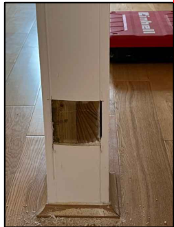
Modern timber post exposed
