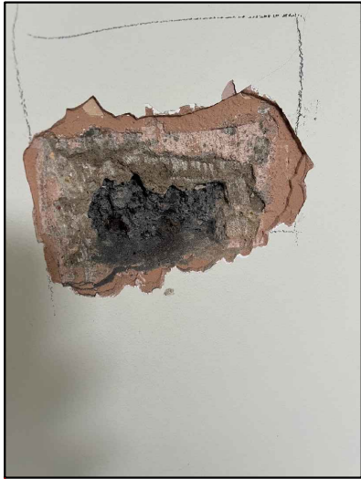
Modern block work
