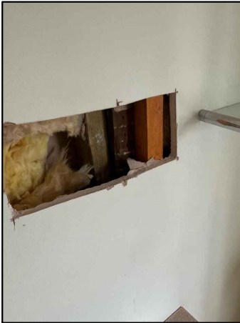
Original and modern timber stud work. Doorway to be created within the frame of original timber stud work; retention of the rest of the wall.
