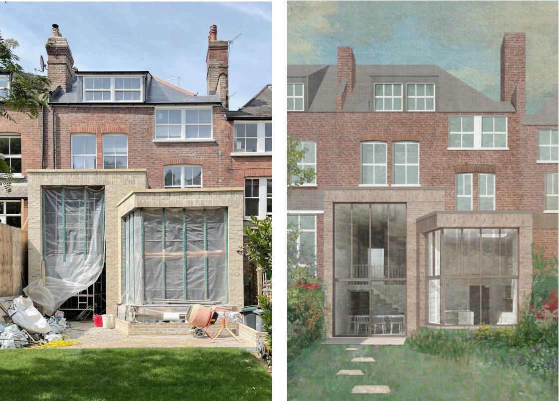
Top - Aerial view of the rear elevations along Talbot Road with No.31 under construction Bottom - Approved rear extension at 31 Talbot Road (HGY/2021/0307), under construction and approved design (image credit Emil Eve Architects)
