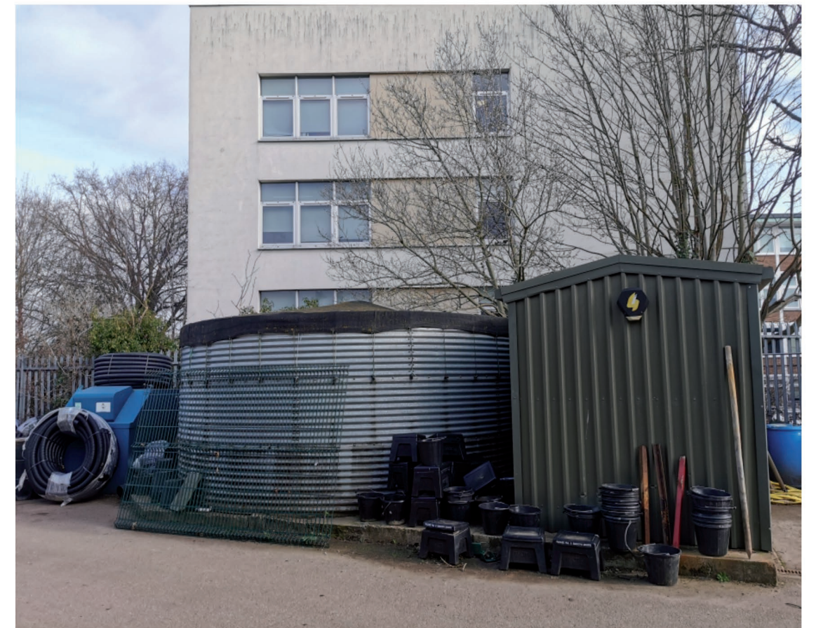
Existing Water tank
