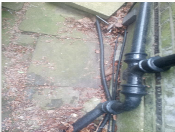
Fig 1.1: Trial Hole 1 Location
