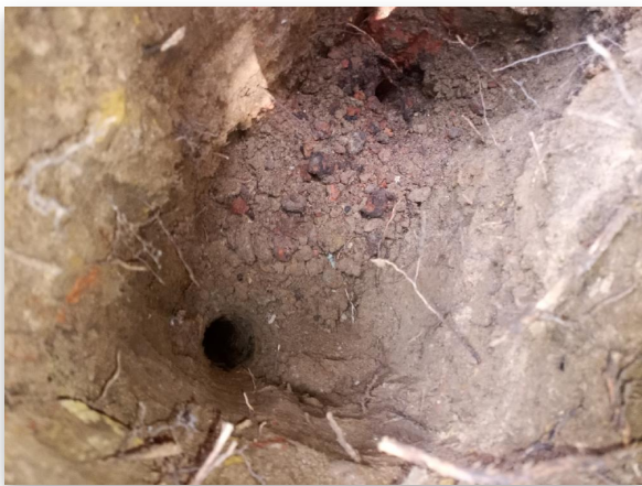
Fig 1.2: Trial Hole 1 Footing
