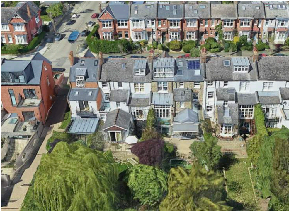
Application site viewed from the south
