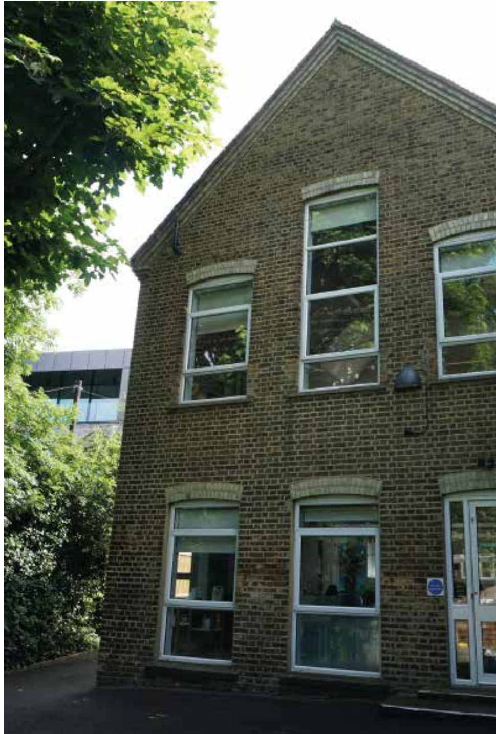
Rear of Infant Building
