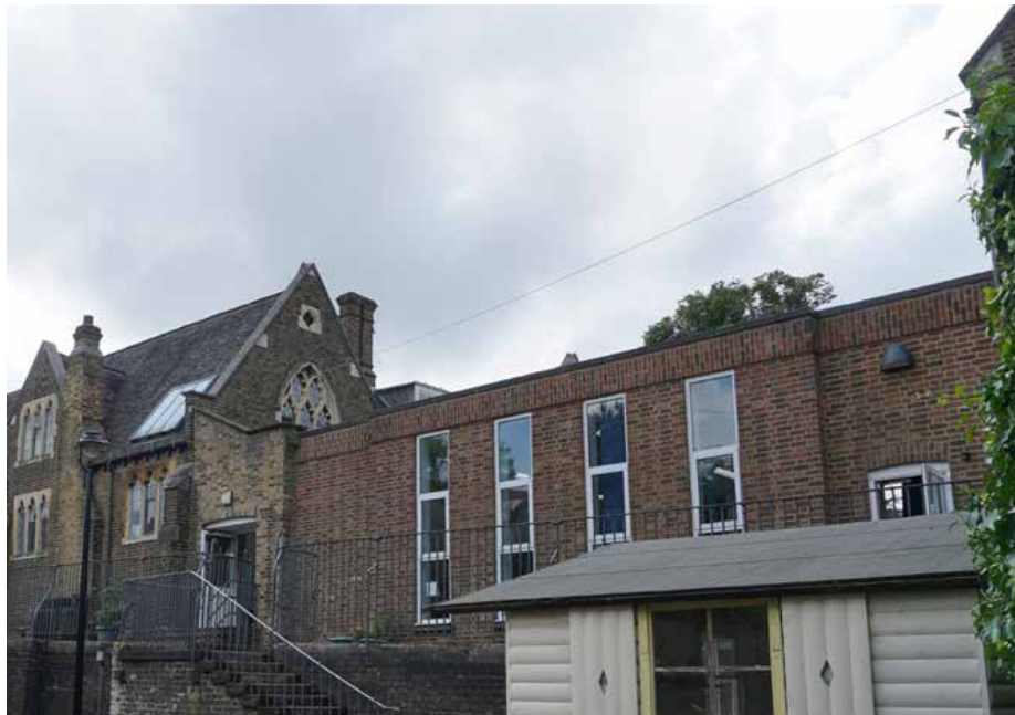
Infant Hall Infill Final architectural intervention 1980
