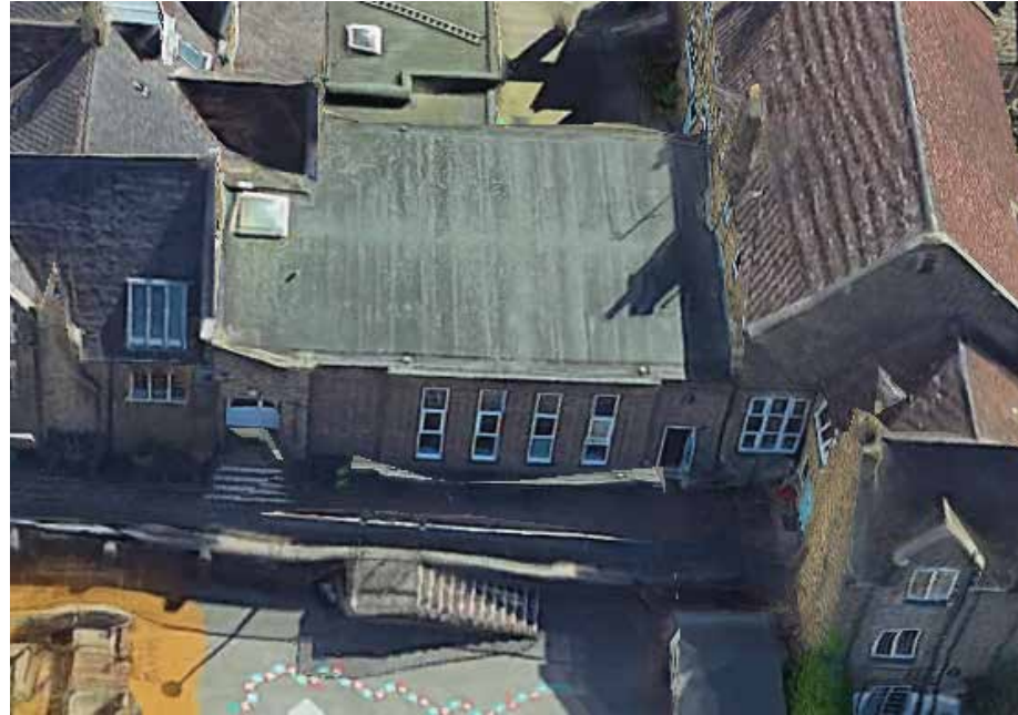
Infant Hall Infill Final architectural intervention 1980
