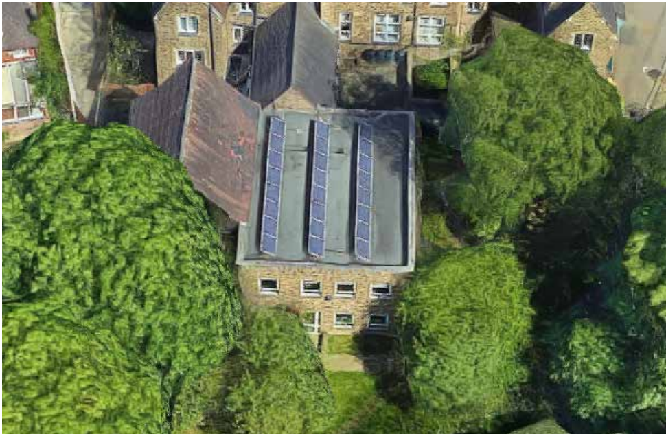
Rear of Infant Building (Aerial)
