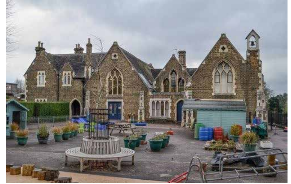
Front of the Site
