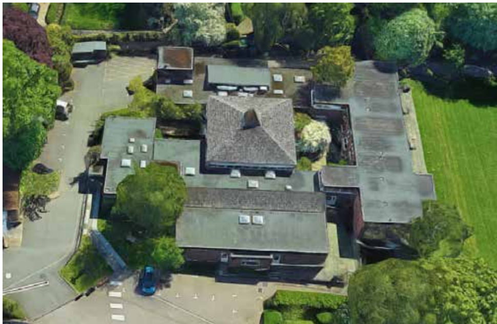
Junior Building Aerial View
