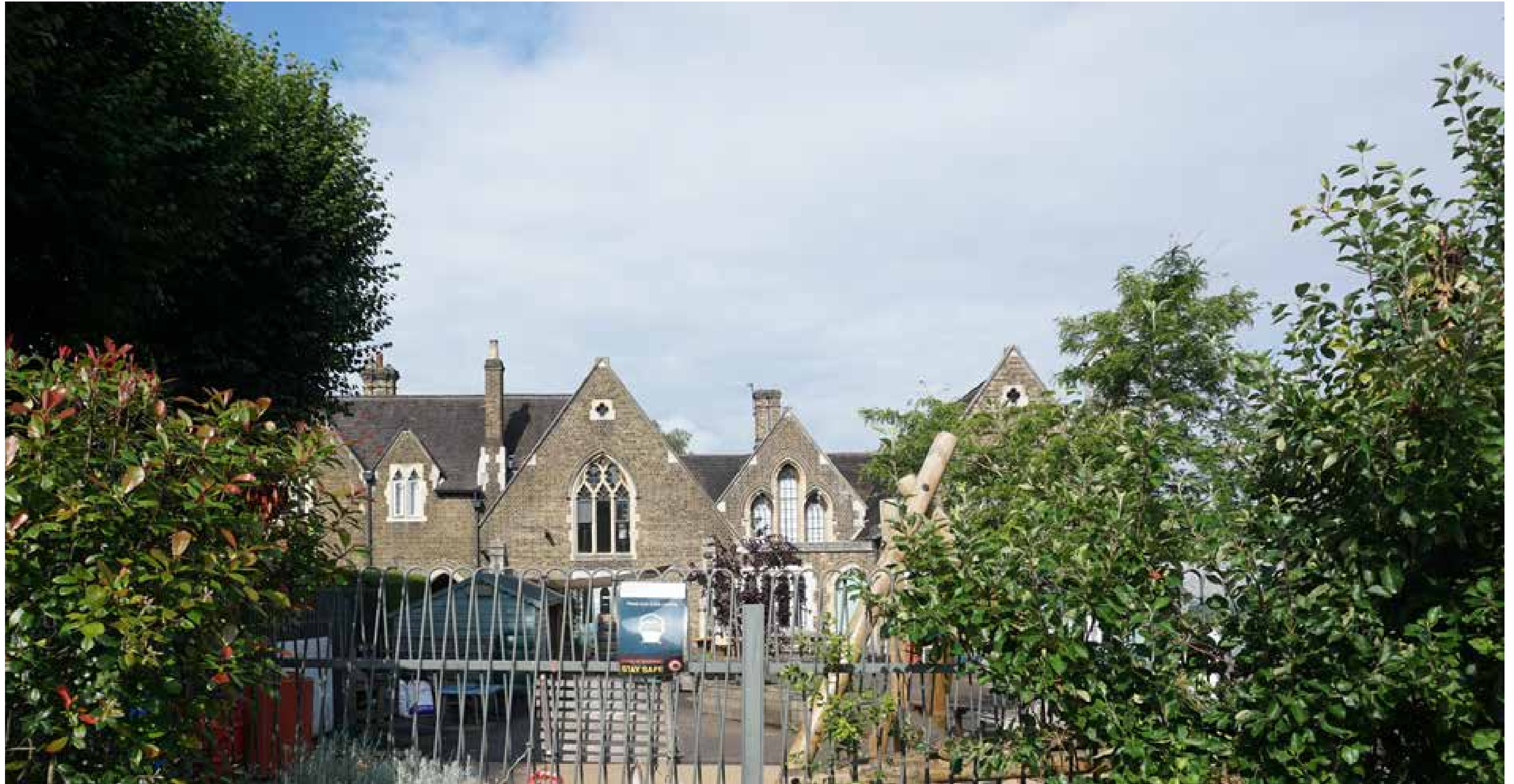
Above: Existing View (Pavement North Road)
