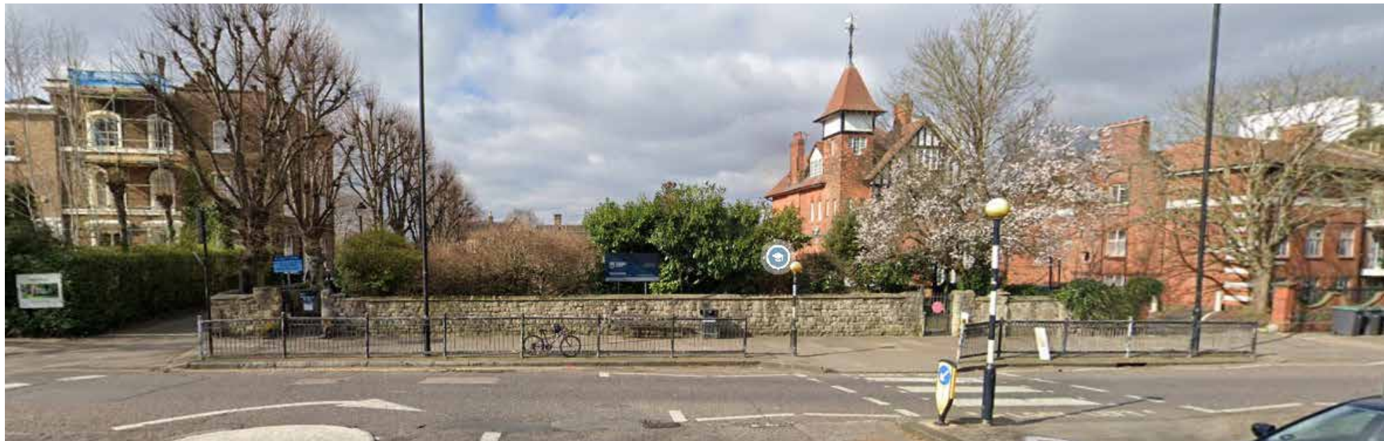
North Road Streetview
