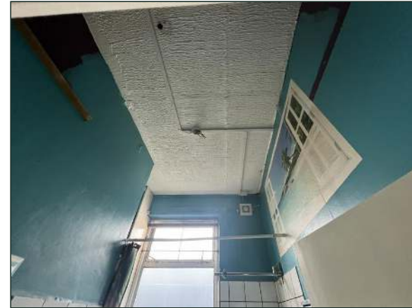
Photo 14 - Flat C Bathroom
