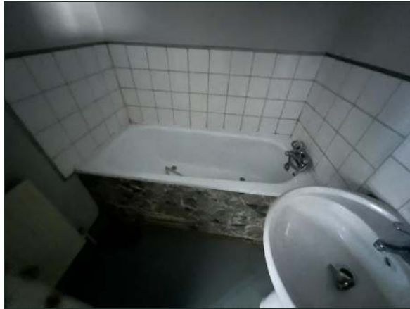
Photo 105 - Flat A - Bathroom
