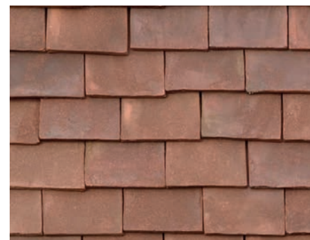
fig.15. Plain clay tile to match existing
