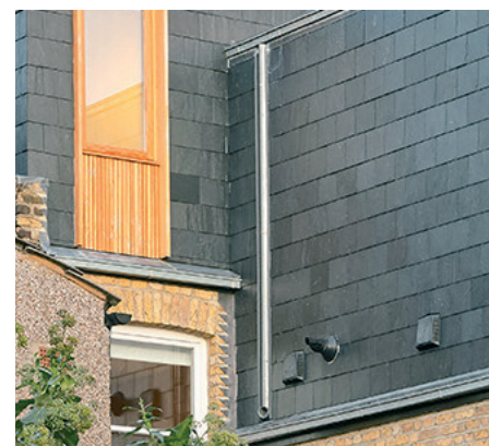
fig.14. Gutter and downpipe flush with tile
