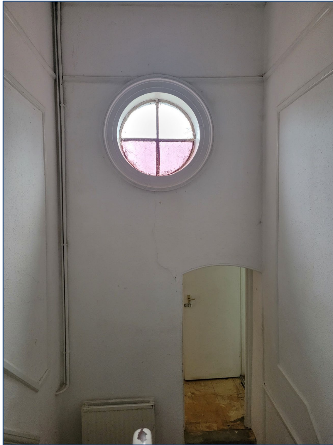
Image 3 Circular window retained visible from rear elevation
