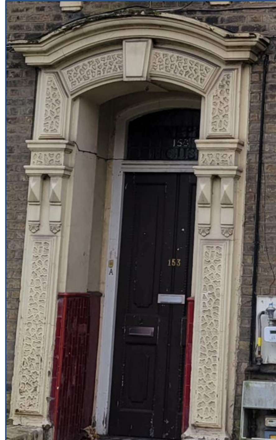
Image 2 Surround detail – one of many
