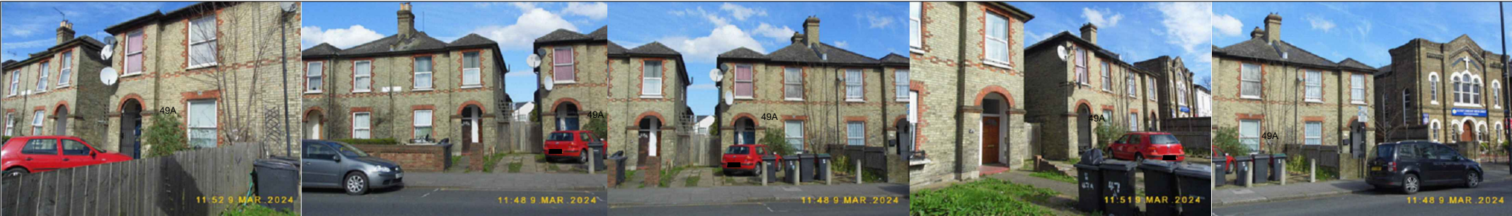
FRONT VIEW LOOKING WEST FRONT VIEW LOOKING WEST FRONT VIEW FRONT VIEW LOOKING EAST FRONT VIEW LOOKING EAST
