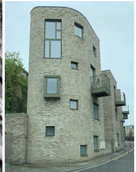
Kiln Place infill housing
