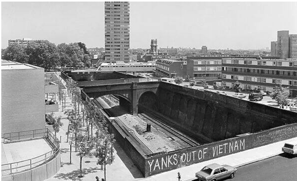
Old Haverstock Hill Station: open cut railway canyon
