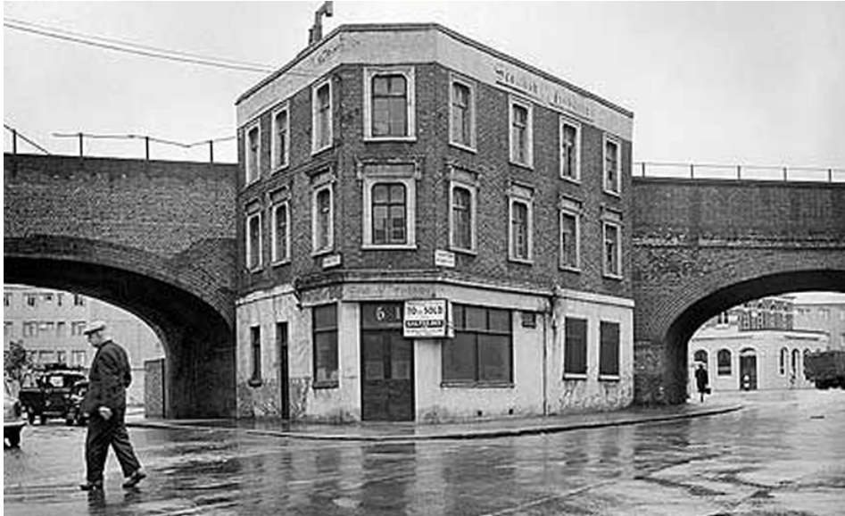
61 Grafton Rd: Interface of housing & infrastructure
