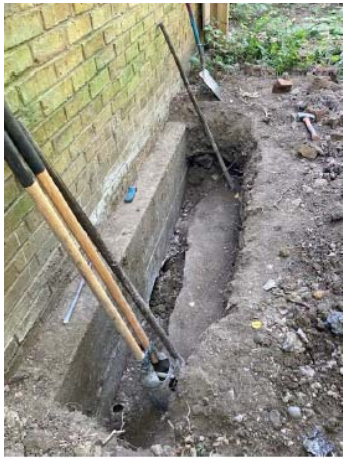
Trial pit along flank wall with neighbour
