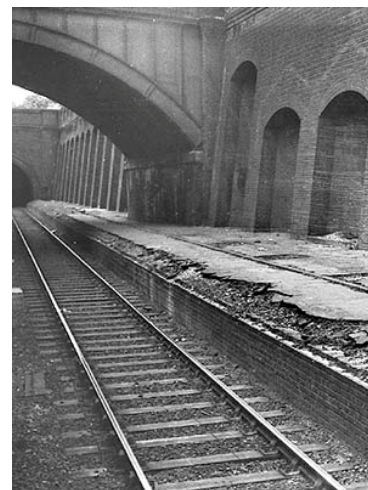
Midlands Railway arches & architecture
