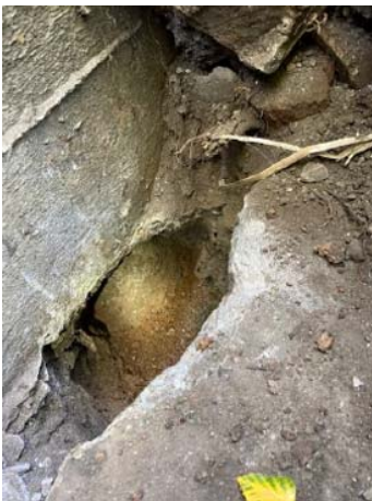
Trial pit along flank wall with neighbour
