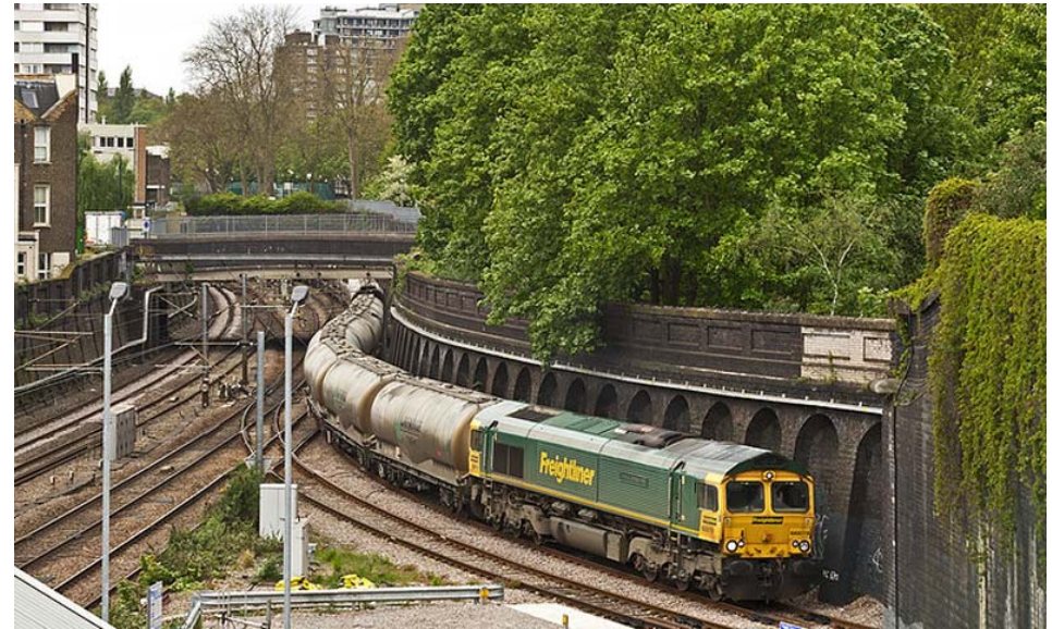
Carlton Rd Junction: Brick embankments & viaducts
