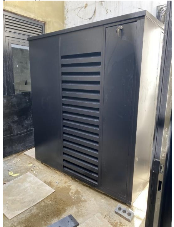
Figure 1– Typical Condenser Attenuated Enclosure
