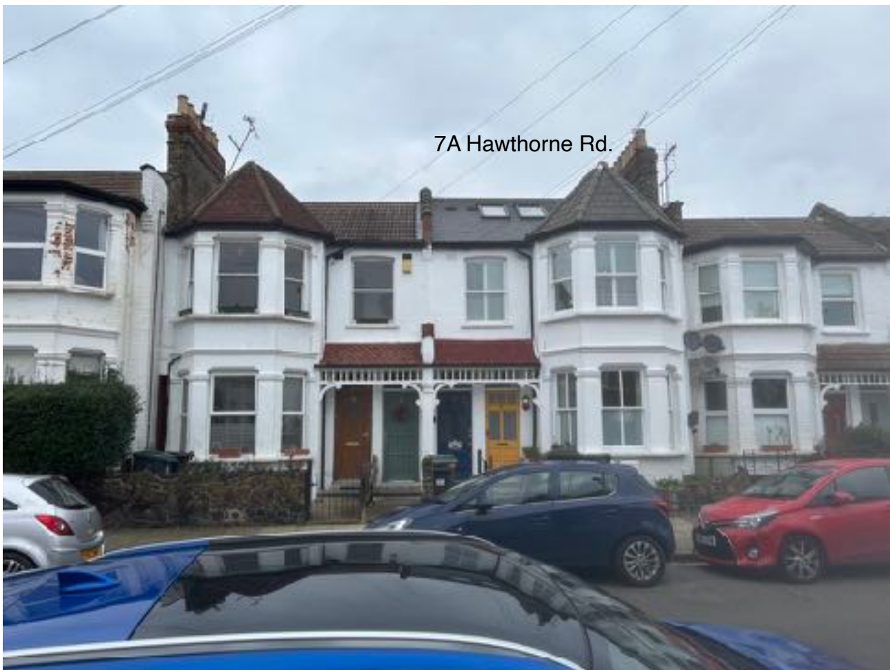
7A Hawthorn Rd. with glazed rooflights to the front main roof. The rear half dormer roof extension is not visible from the road
