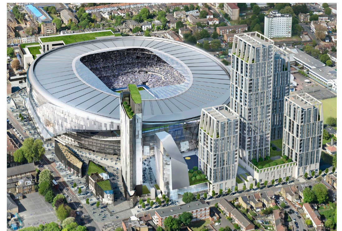
FIGURE 42. Aerial View of the Stadium Southern Development
