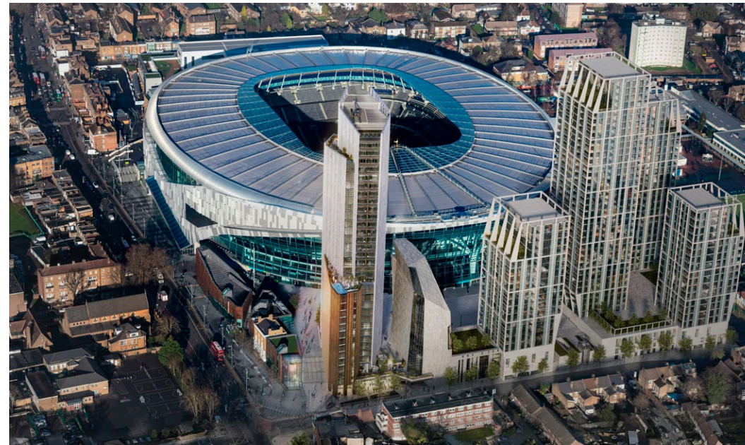
FIGURE 43. Southern Development Aerial Overview
