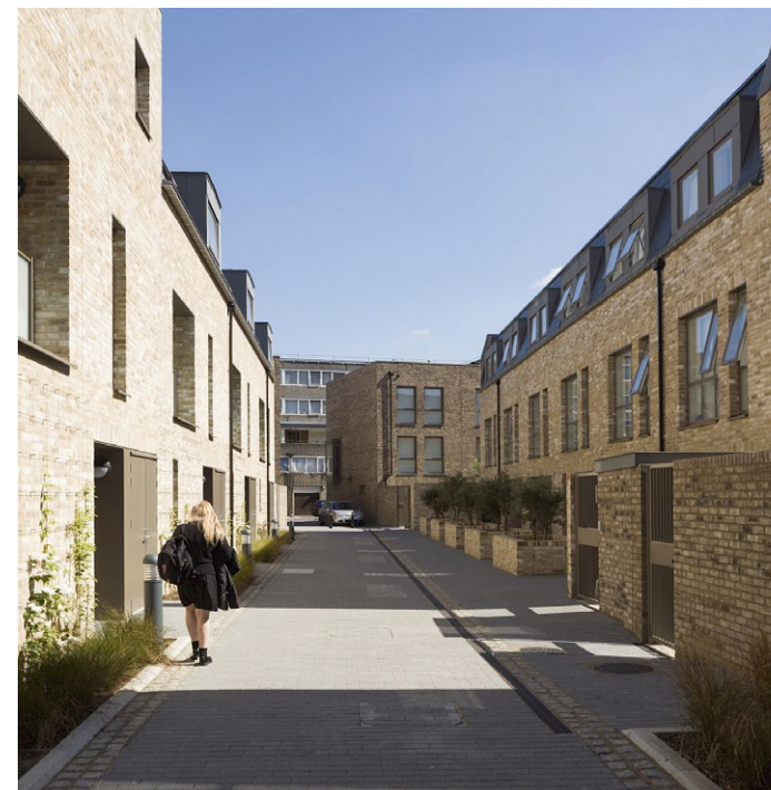
FIGURE 71. Shared surface road. Alesbury Estate (Southwark) by PTE Architects
