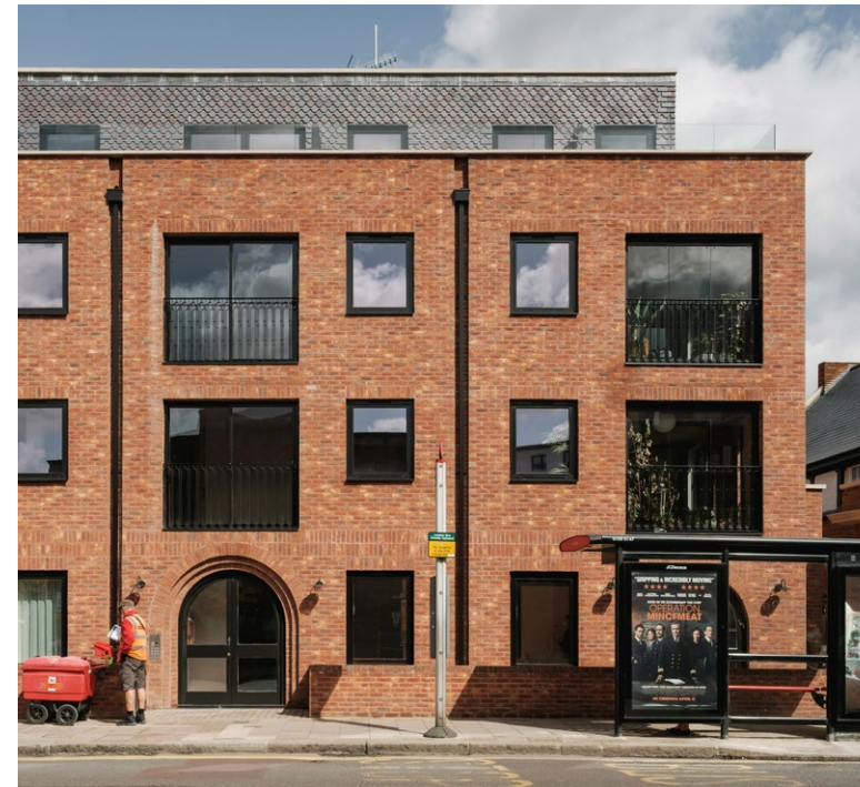
FIGURE 67. Residential development (Harrow Road) by GPAD
