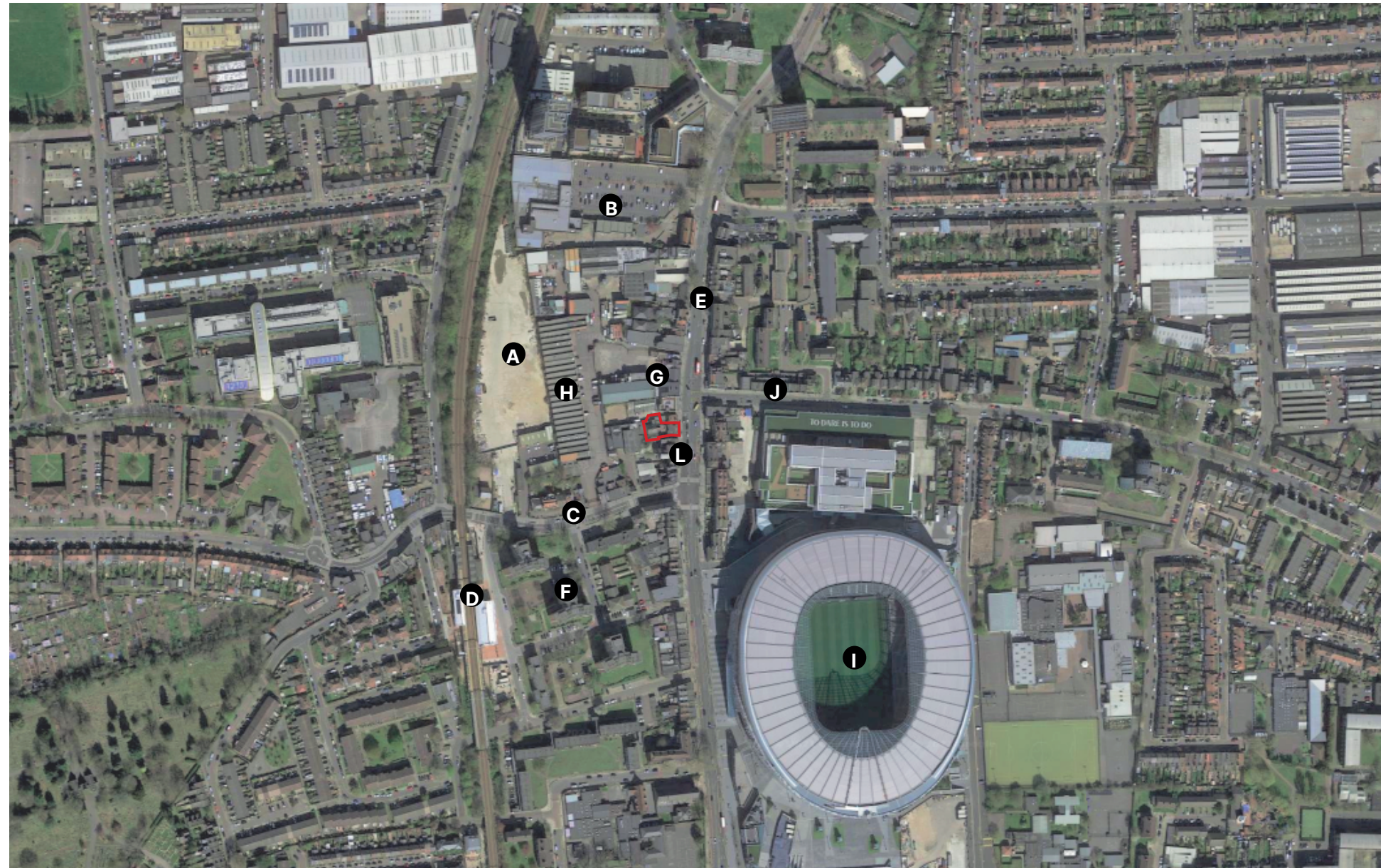
FIGURE 1. Site Aerial Overview
