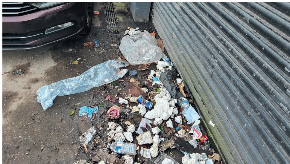
Partially blocked drain and back storage area access
