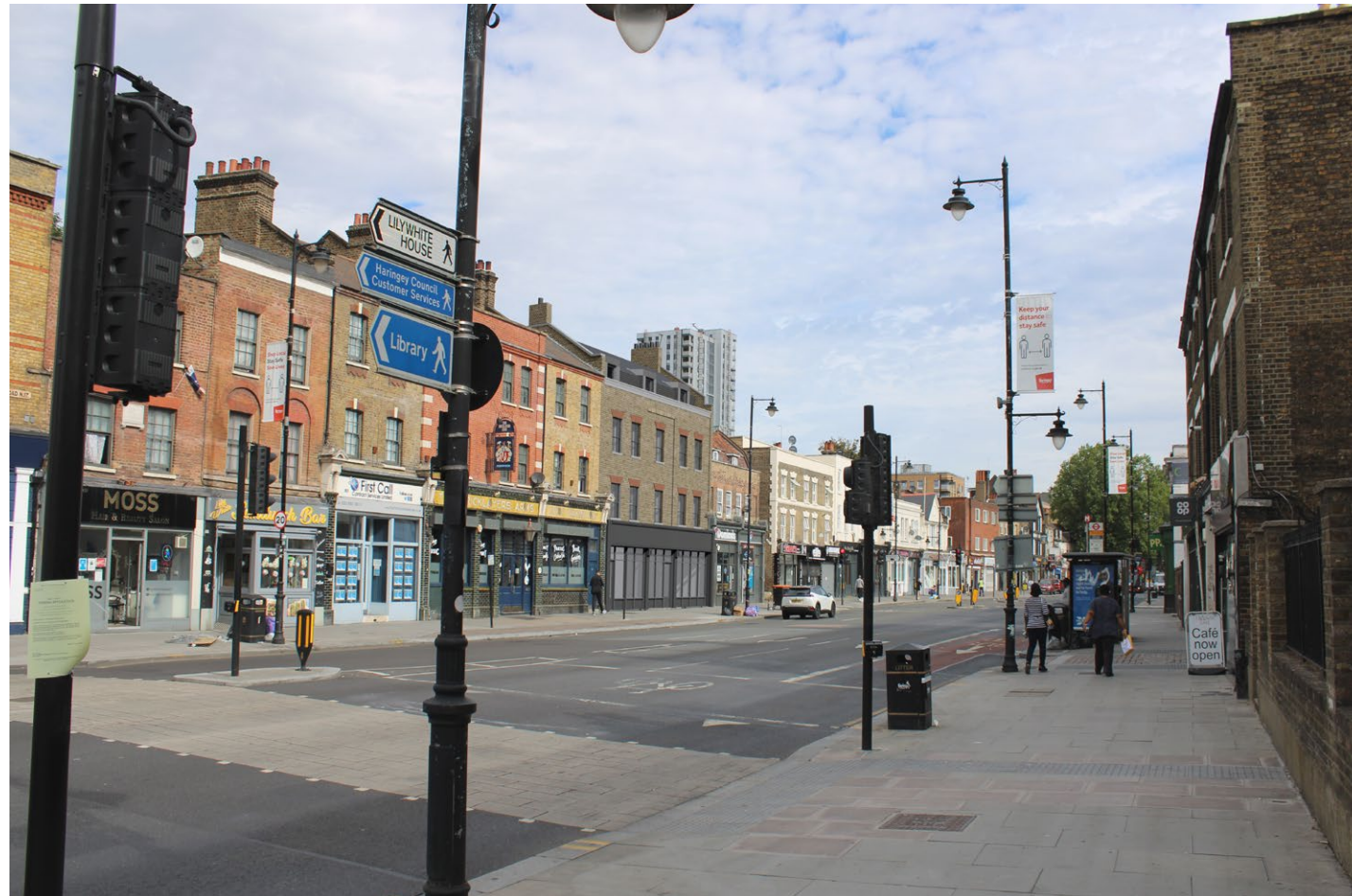
FIGURE 73. View north from High Road eastern foot way
