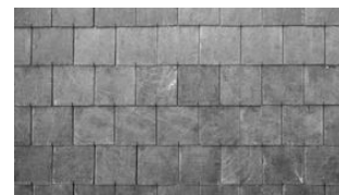
1. Slate tile roof
