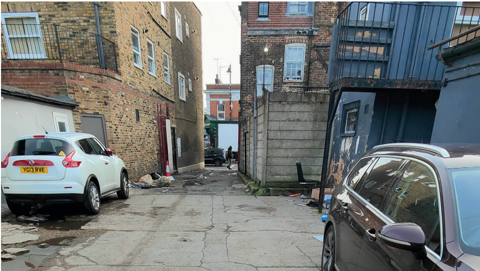
Alleyway (Percival Court), access to north side of building
