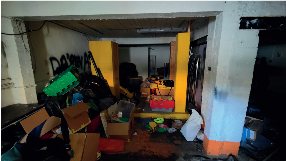
Inside of back storage area, used for storage of sports equipment
