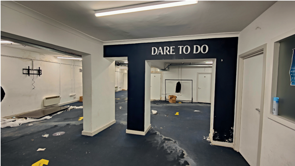
Ground floor of building, with access to meeting rooms and toilets
