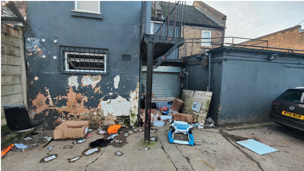
Fly tipping at north side of site
