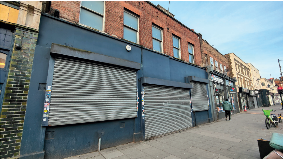
Front of building at east side of site
