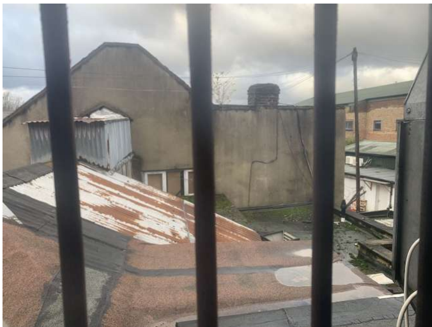
Plate 4 - Single storey extension (foreground) and two storey annex (background) looking east from second storey of terraced building
