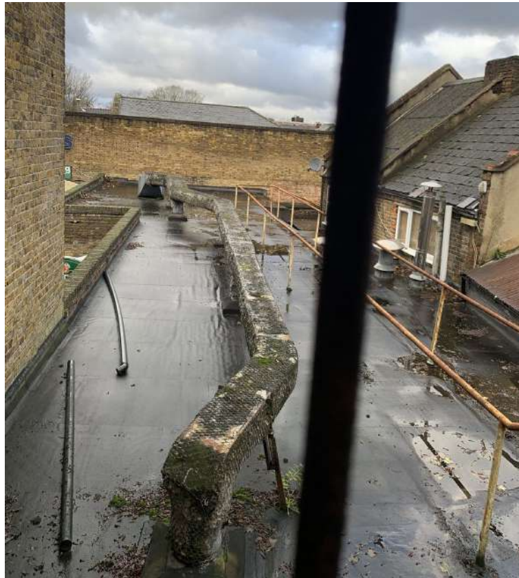
Plate 3 - Single storey extension looking east from second storey of terraced building
