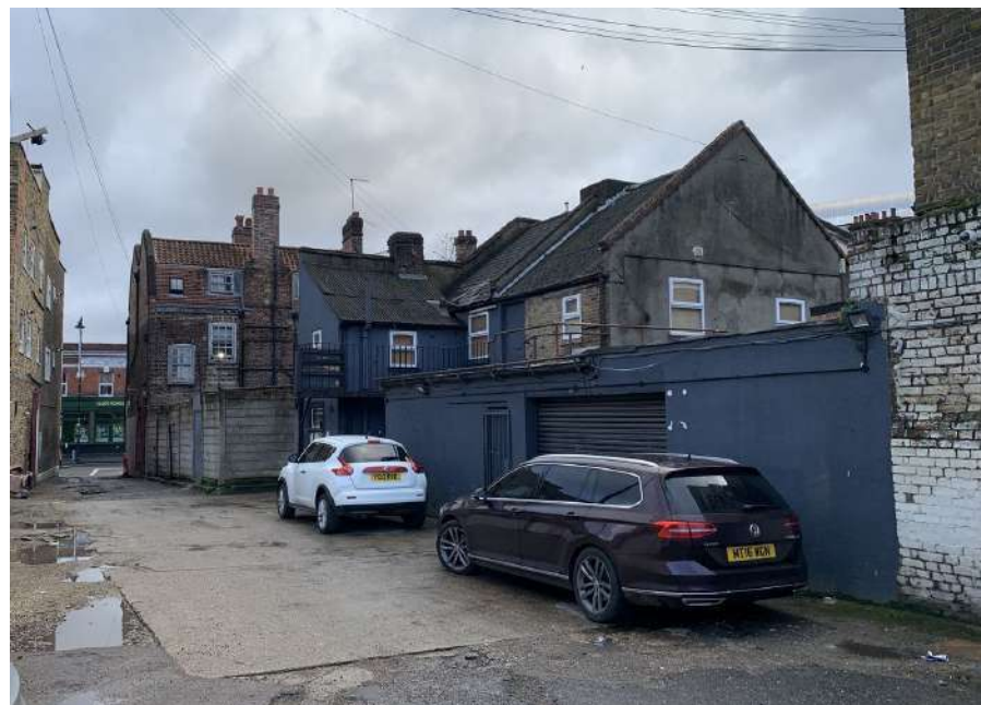
Plate 2 - View of northern boundary of site along Percival Court looking east
