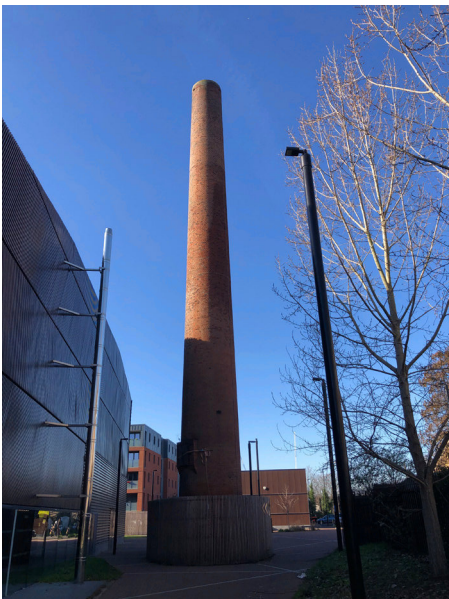
The chimney of previous public baths
