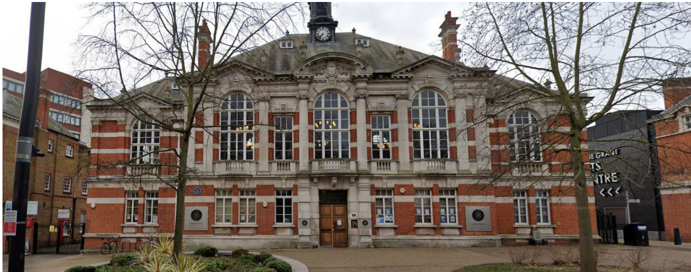
10 - Former Town Hall along Town Hall Approach road
