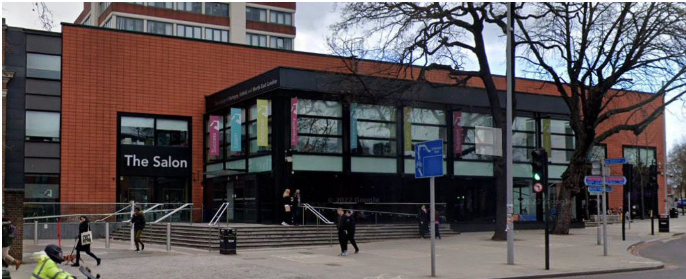
8 - CCCG Centenary Building - Main Entrance for College.
