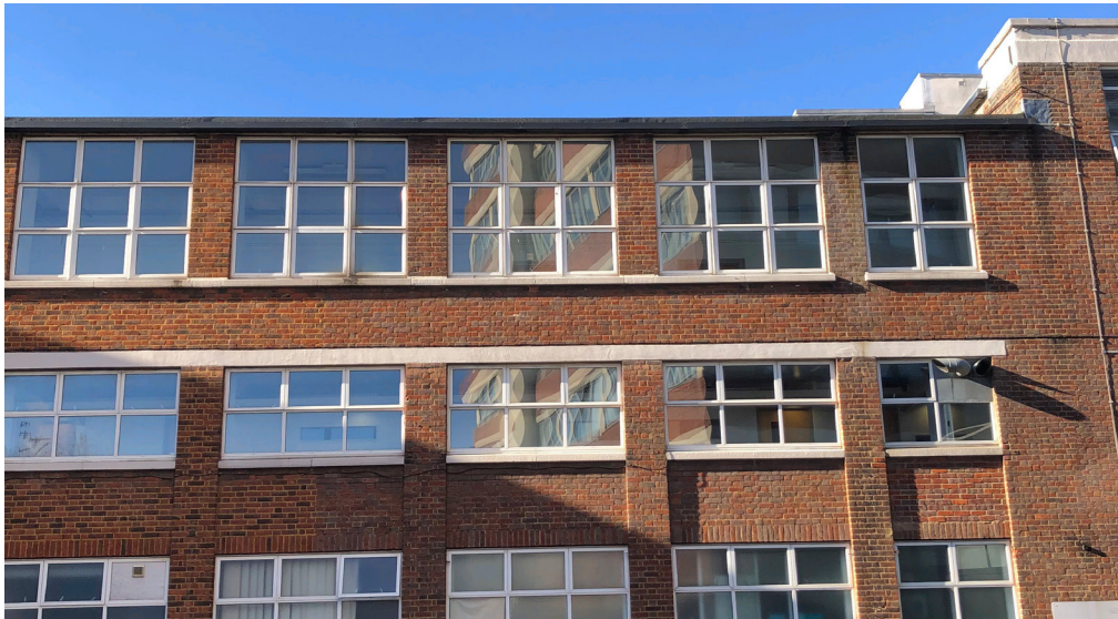
11 - Existing College buildings to rear and centre of campus
