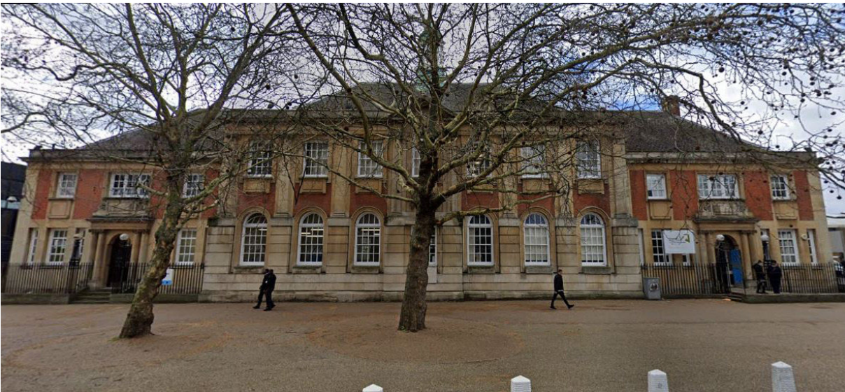
3 - The College of North East London along Town Hall Approach road
