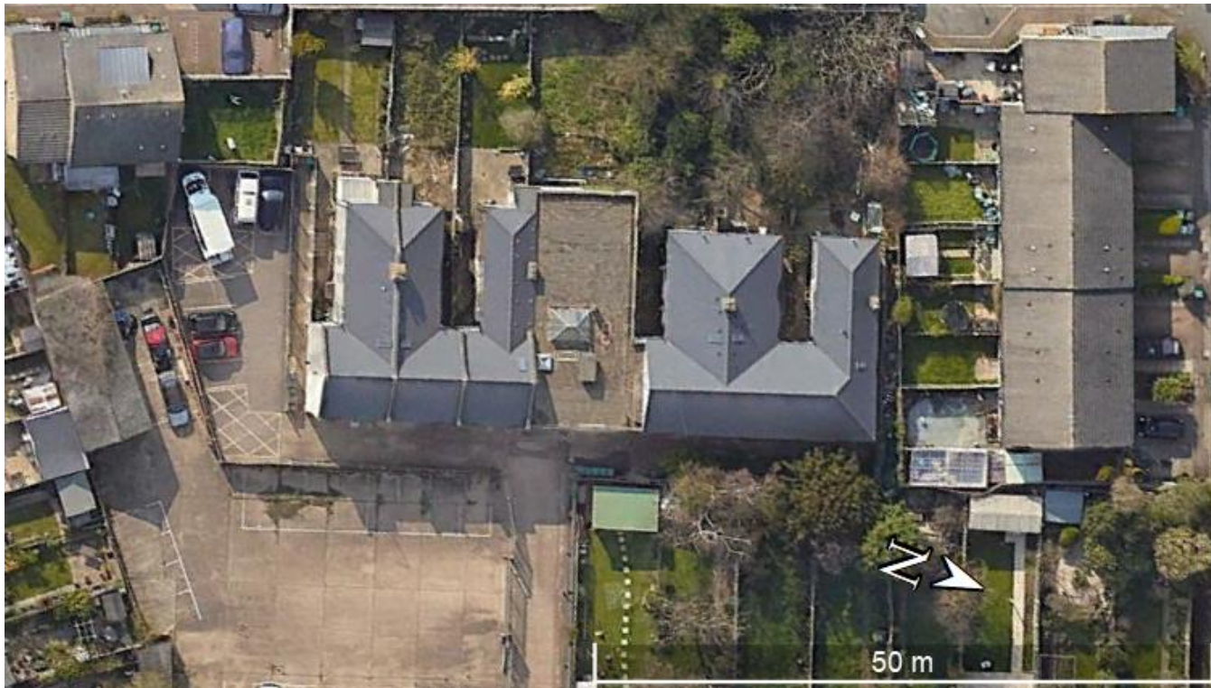
Figure 1-1 – Frederick Morfill House site
