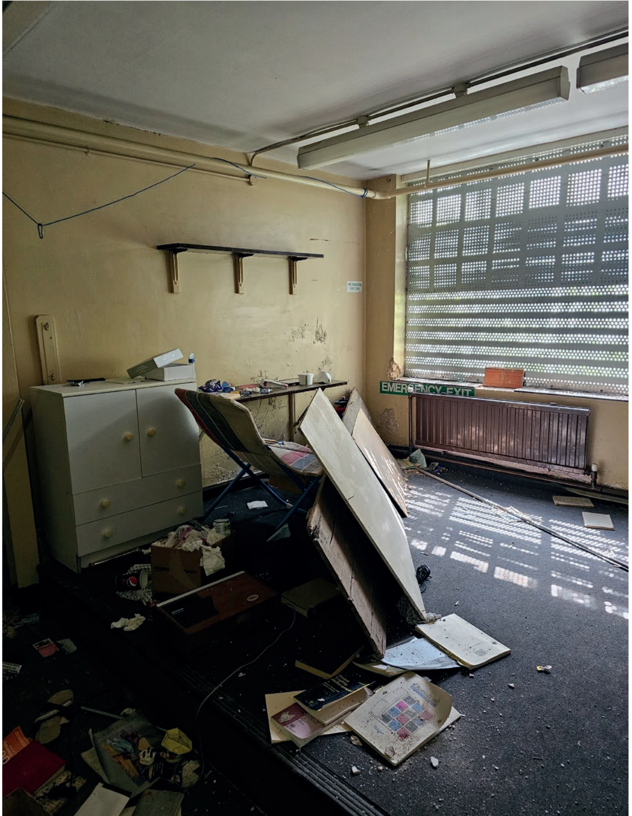
Internal view of the main office space to the front of the building
