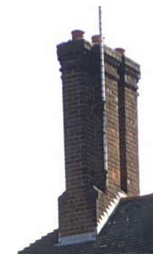
Guildens original decorative brick chimney
