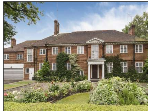
ORIGINAL FRONT FACADE - GUILDENS
