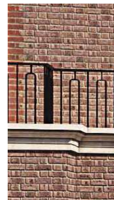
Local example of black cast iron railing
