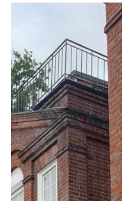
Black metal railing featured on front terrace at 14 Templewood Avenue
