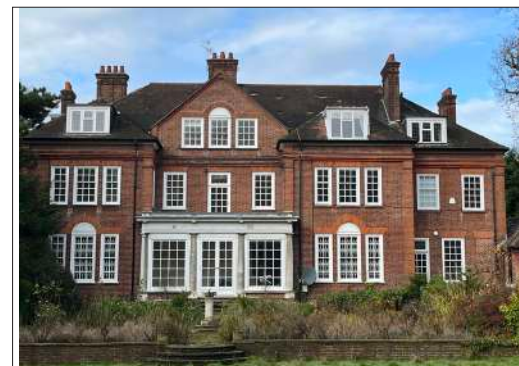
REAR OF 14 TEMPLEWOOD AVENUE - QUENNEL
