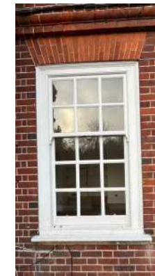
Sash vertical sliding windows seen at 14 Templewood Avenue, with Flat arch splayed course brickwork
