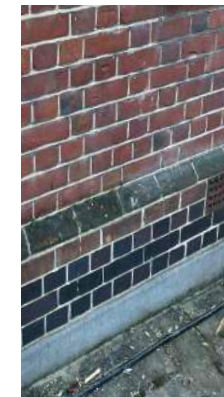
Extruding brick plinth featured on 14 Templewood Avenue
