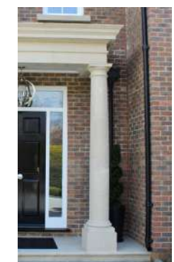
Tuscan styled stone columns with stone cornice, frieze and fascia
