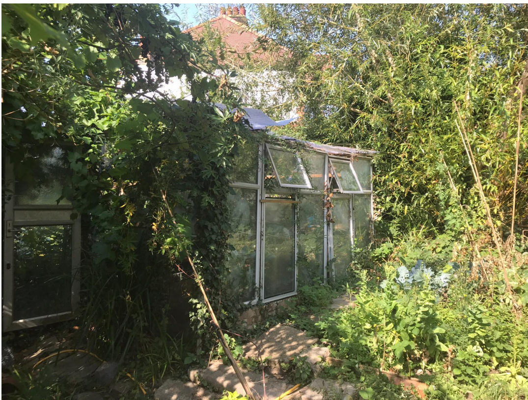
Photograph 8 – Concrete tiles/slabs located around the perimeter of the derelict greenhouse.
