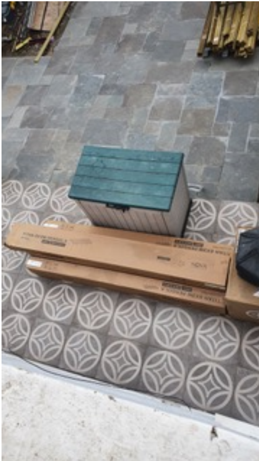
Use of unsuitable materials for historic Edwardian house in Conservation area
