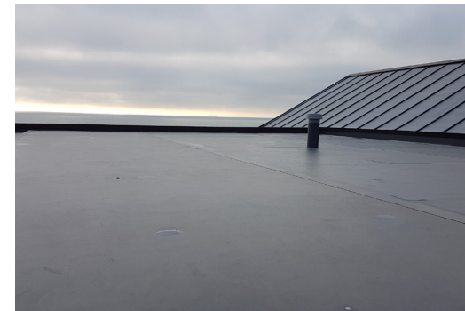
Renolit Single Ply Membrane- salmonsolutions.co.uk
