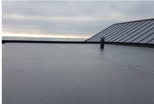
Renolit Single PLY Membrane- salmonsolutions.co.uk
