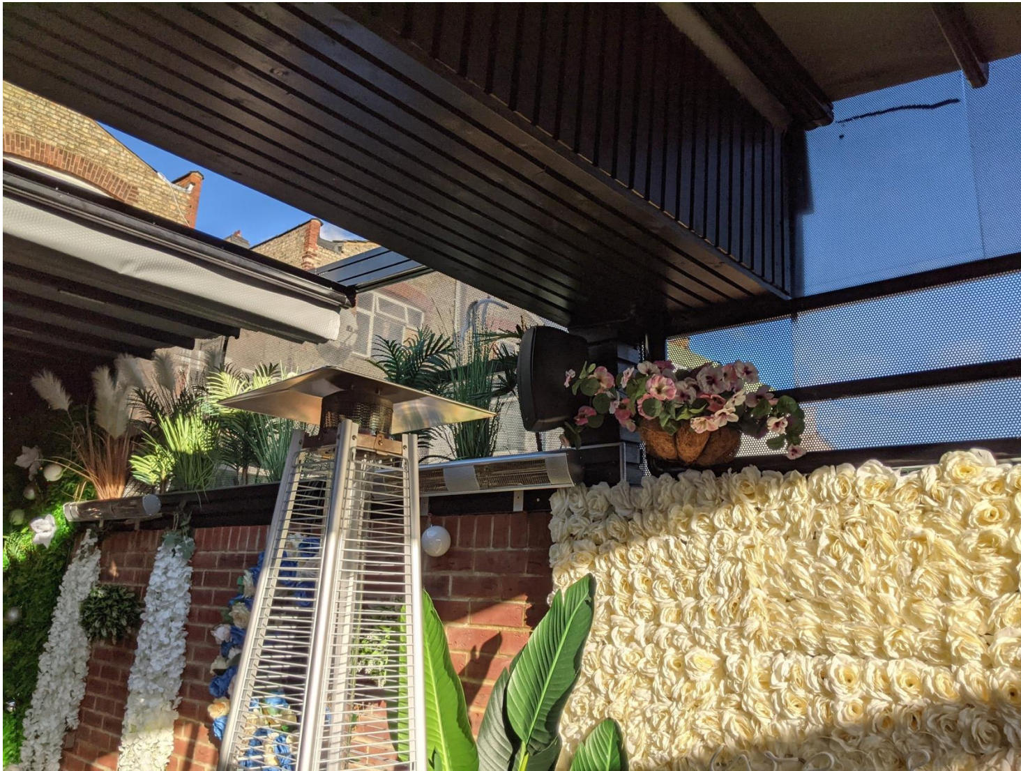
Moon Resto Lounge, 34 Hornsey High Street, N8 Internal View Showing Lightweight Roof and Ventilation Project 13212
